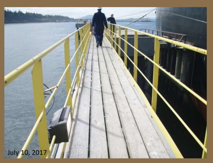
Replace solid wood surface on walkways with grating and 60% light penetration.
