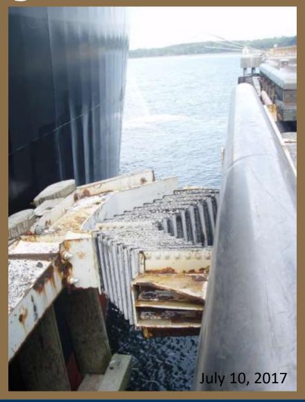
Replacing steel whale on north fender and rubber elements on the fenders.
