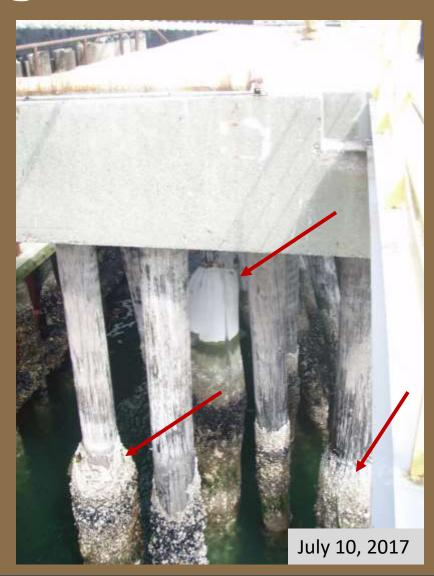
Pilings shown in this photo have been encased with grout.
