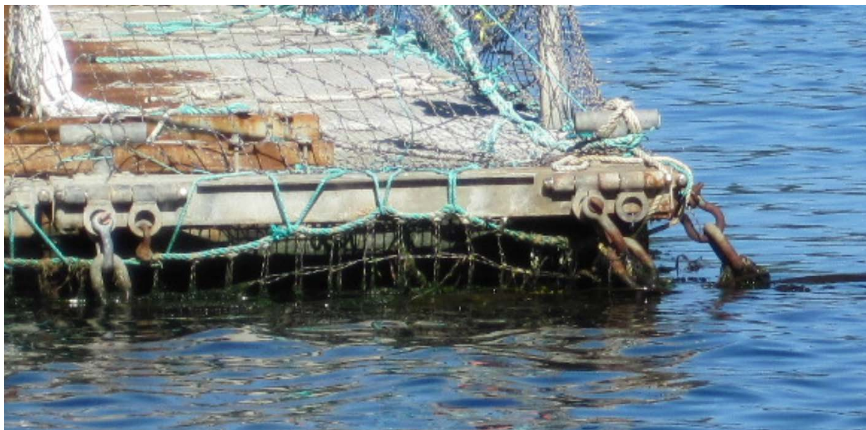
Figure 6. Corner of Cypress net pen #1 on September 30, 2016, showing pad eyes on hinges on side of steel platform (“outrigger” section). Shackles connect anchor chains to pad eyes. Design and configuration of moorings of net pen #1 same as for net pen #2.
