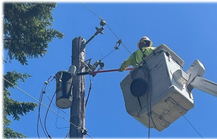
Figure 1 - Overhead Transformer Installation
