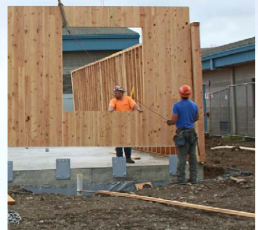
Cross laminated timber project building at Greywolf Elementary in the Sequim School District.
