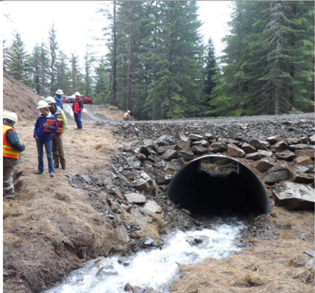
Figure 3. Mainline Fish Blockage repaired with a new better crossing
