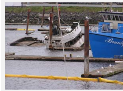
Figure 1: Photo showing damage and recovery efforts in Crescent City Harbor shortly after the March 11, 2011 tsunami (Credit: Rick Wilson).
