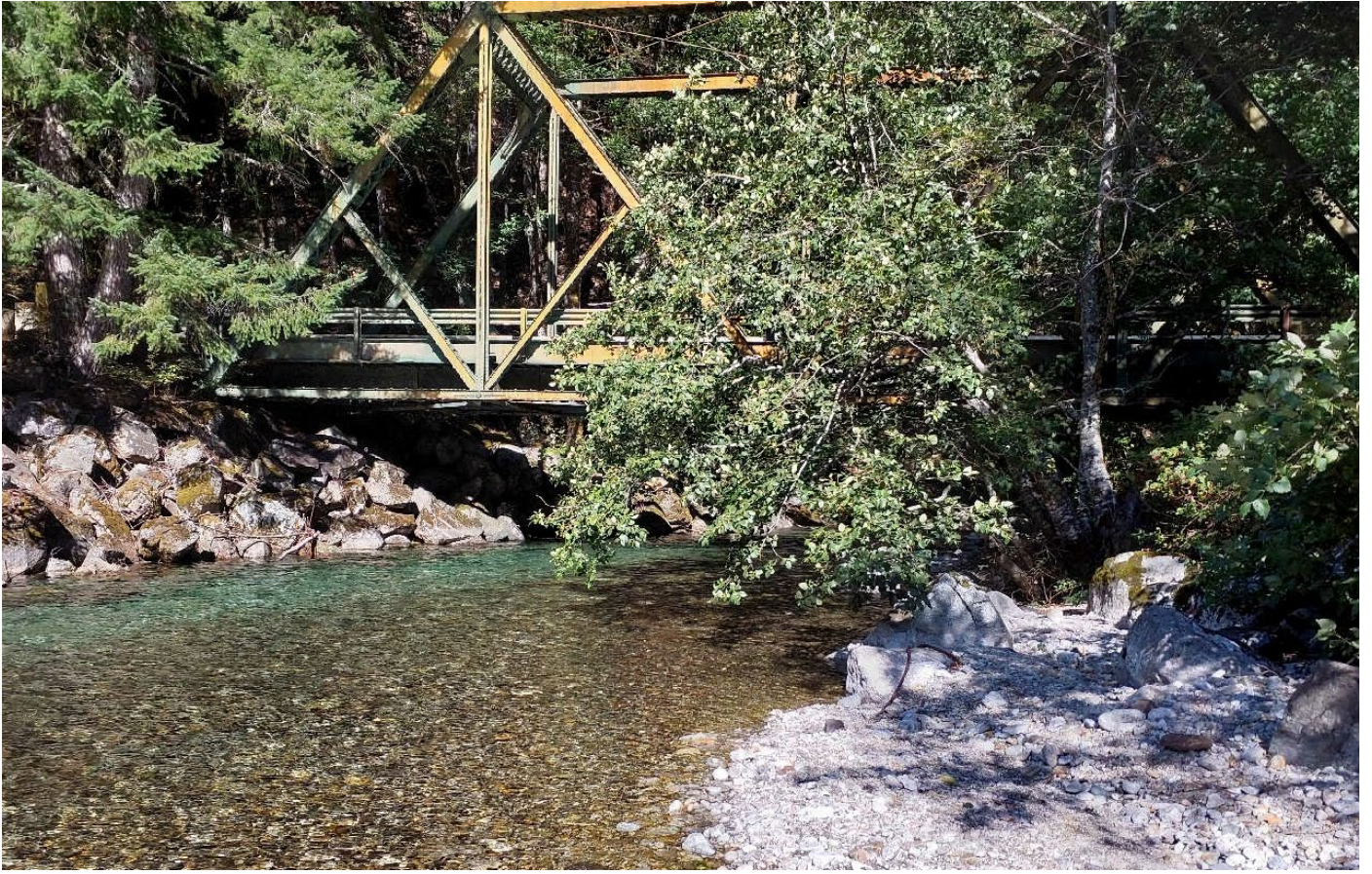
Figure 2. Stetattle Creek bridge, looking upstream.
