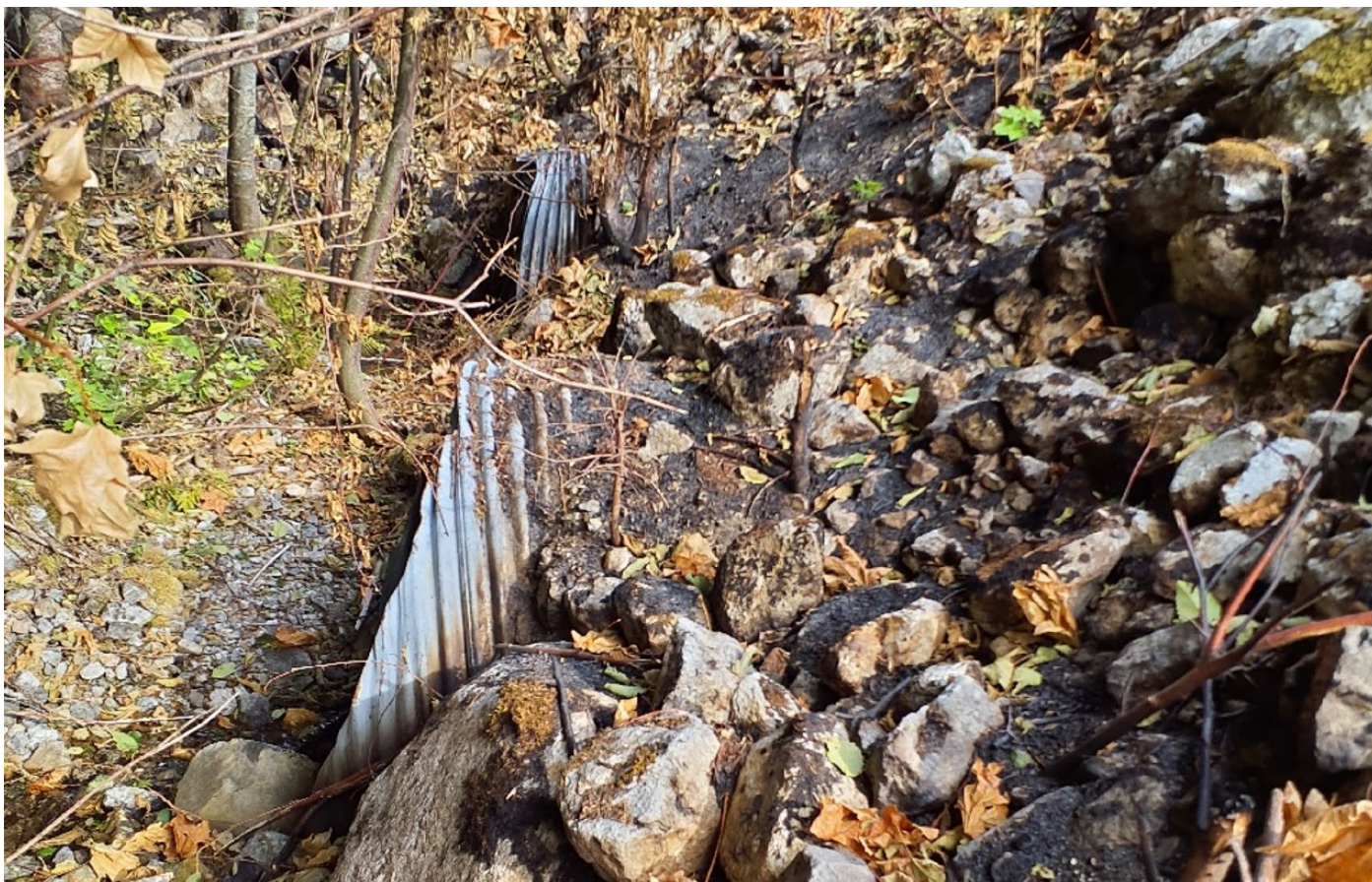
Figure 1. Inlet side of culverts at Sourdough 1, looking east.
