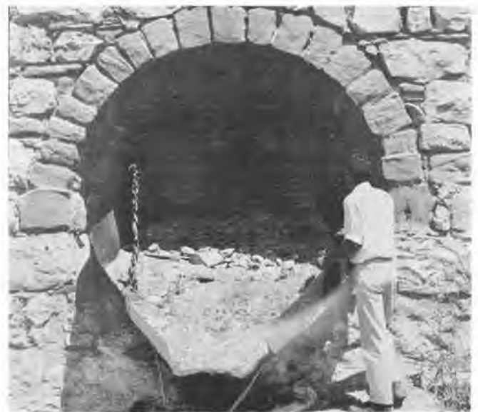
FIGURE 13.—Opening at base of limekiln for removal of lime. Cowell quarry, San Juan Island, San Juan County.
