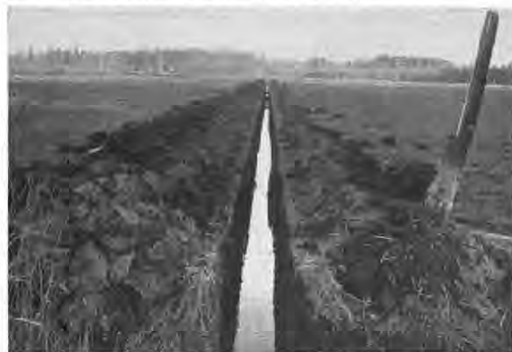
FIGURE 185.—Hand-dug drainage ditch in woody peat on farms of J. Sesby and C. French, 4 miles southwest of Arlington, U. S. Department of Agriculture Soil Conservation Service photo.
