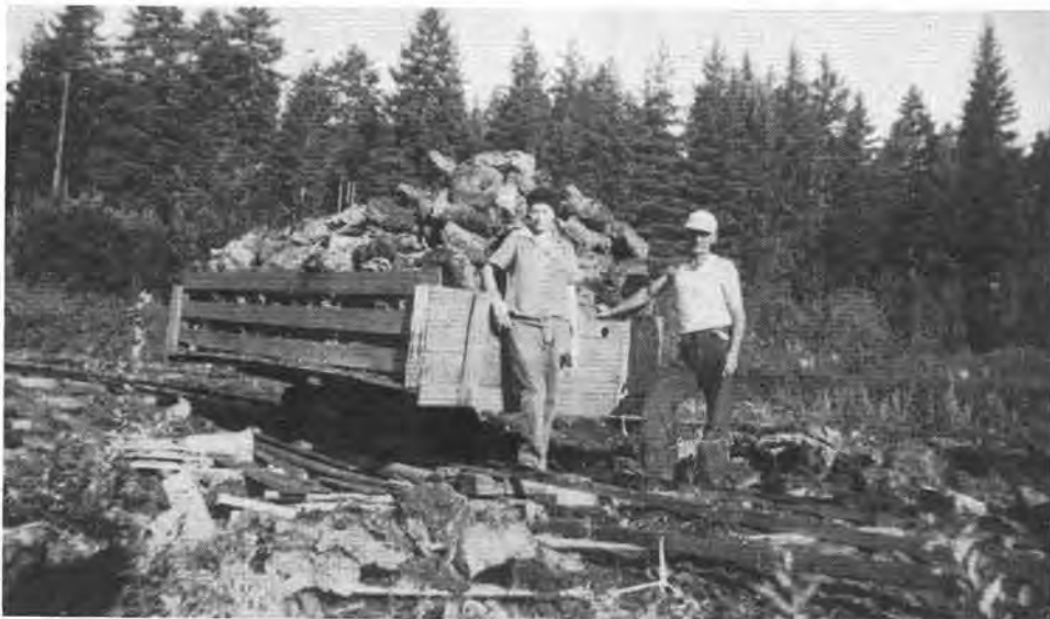
FIGURE 85.—Hauling excavated blocks of sphagnum moss from bog to storage shed on handcar, Tahuya Lake peat deposit.
