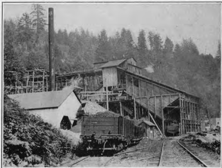
A—Bunker at Grand Ridge Mine.
