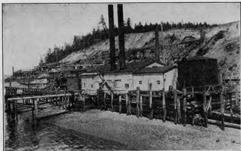
Plant of the Pioneer Sand and Gravel Co., Stellacoom.
