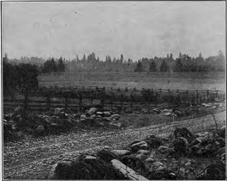
A gravel outwash plain in Thurston County, and a highway constructed on it by the removal of the coarse material.
