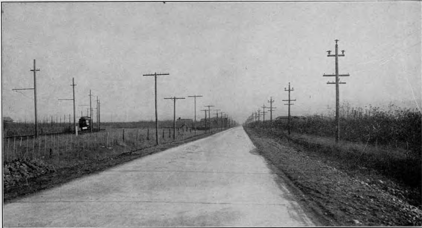
The Apple Way, east of Spokane. A concrete pavement whose mix and aggregate were tested by the field concrete cylinder test and abrasion test.
