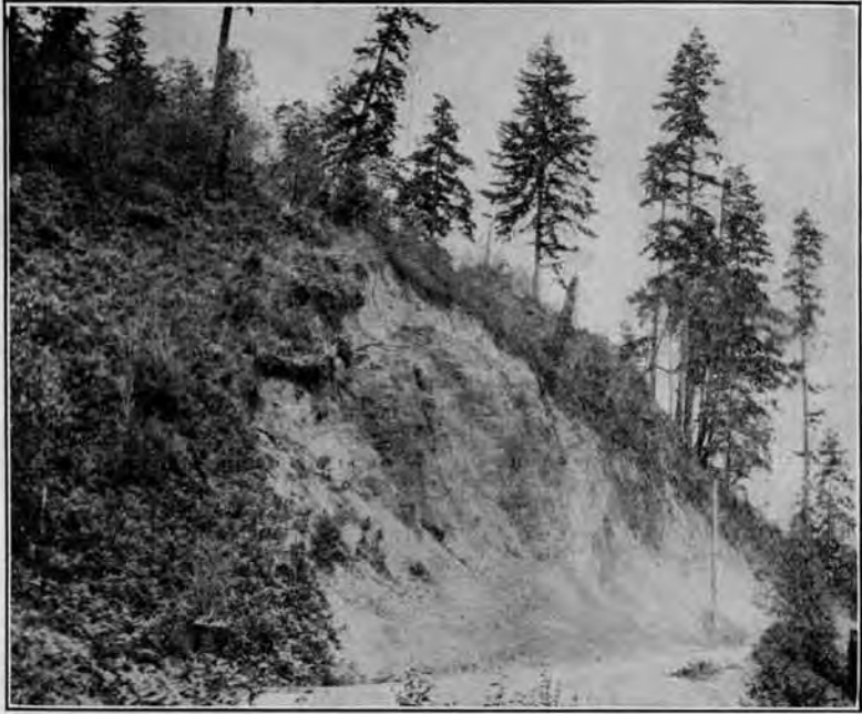
A Gravel Pit used without stripping away the soil. Such gravel is bound to contain organic matter harmful both to cement concrete and to roads gravelled with this material.
