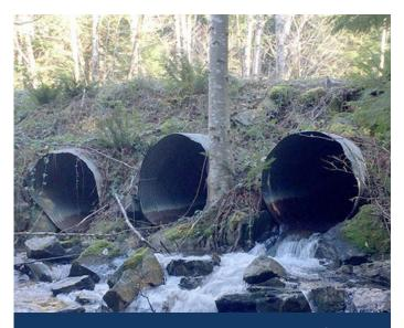
Culverts must be designed in ways that allow fish passage. The Snohomish Watershed includes at least 1,200 culverts that are barriers to fish.
