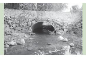
Replacing culverts so they allow fish passage (like this one does) can open up many stream miles of fish habitat across the state.
