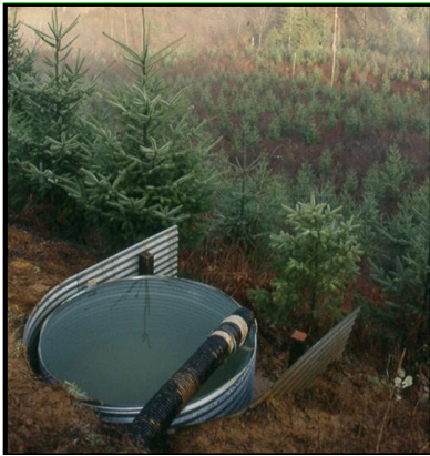
589 590 591 Figure 2: A sediment trap installed below a road segment.
