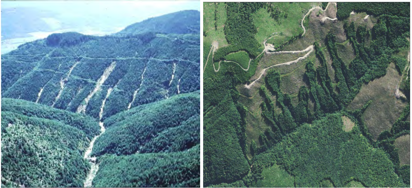
Figure 4. Left: Road-initiated debris flows in unstable landforms, Sygitowicz Creek, Whatcom County (Photo: DNR 1983). Right: Same hillslope 28 years later (2011 aerial photo).
