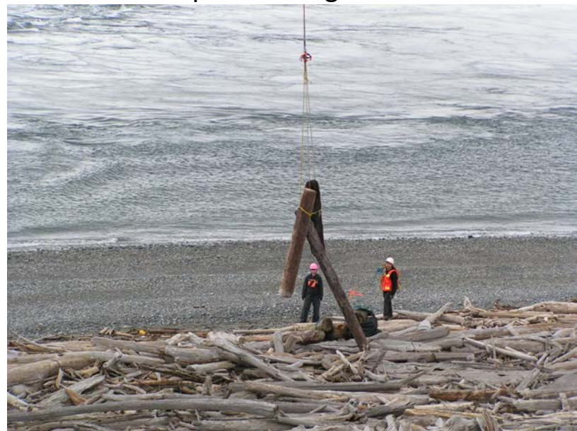
Above: Crawler crane positions logs Below: Helicopter lifts logs off beach
