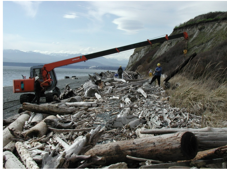
Above: Crawler crane positions logs Below: Helicopter lifts logs off beach
