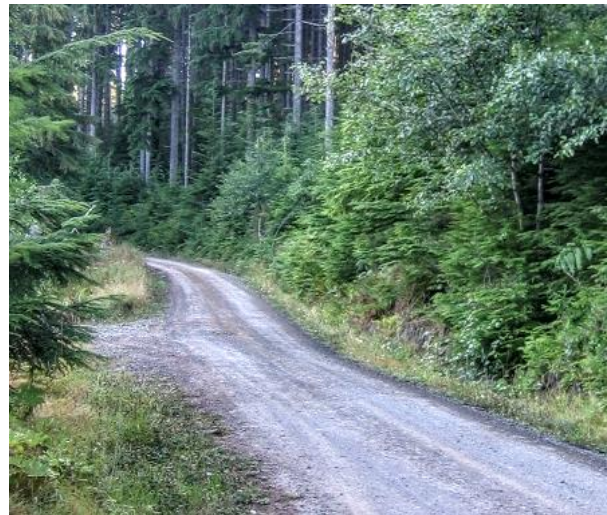
Standard best management practices to minimize erosion include placing crushed surface rock on roads
