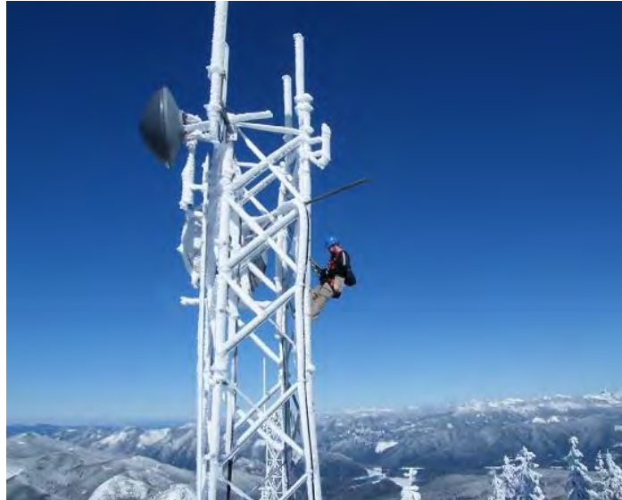
A Technician Repairs Microwave Dishes on a Communication Tower Located on State Trust Lands (Grass Mountain, South Puget HCP Planning Unit). Photo: Steve Diamond/NorthWest Tower Engineering, Inc.
