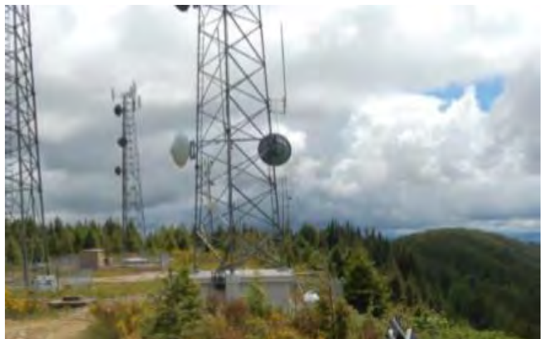
The Radar Ridge Communication Site in Pacific County (South Coast HCP Planning Unit). Photo: DNR
