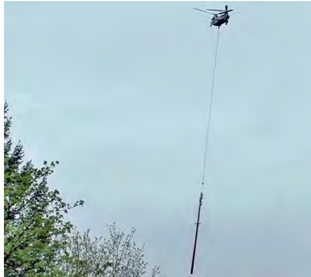
Chinook Helicopter Transports a Replacement Structure to a Remote Portion of a Transmission Line Photo: Bonneville Power Administration
