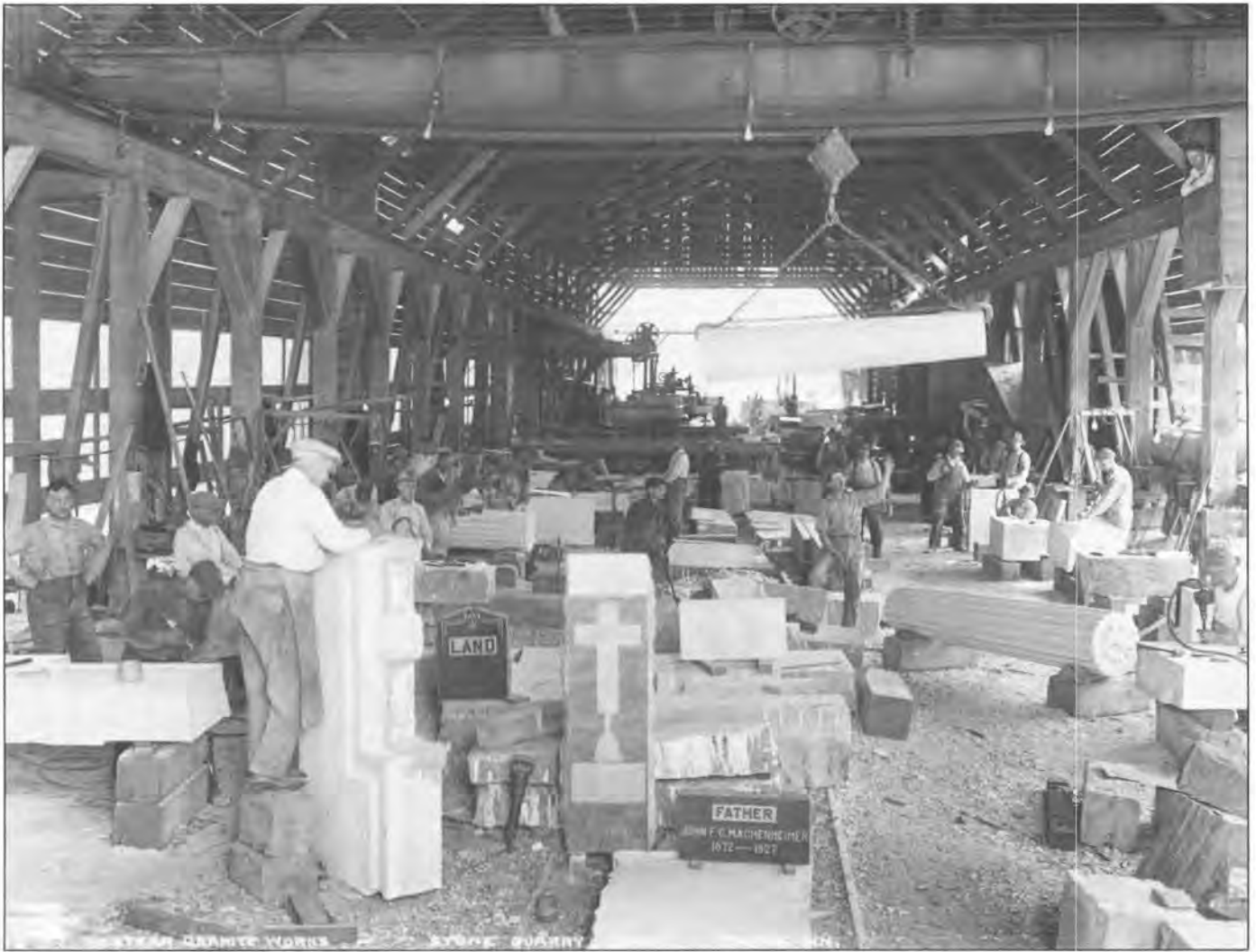
Figure 4. Western Granite Works mill at Index (Soderberg quarry, ca. 1927). Stonecutters finished Index granite and imported stone for buildings and monuments. An "endless chain" holds the suspended column with hooks inserted in holes cut into the ends of the stone (see the column on the right of this photo). Only metal hammers and pneumatic hand chisels were used here because of the hardness of granite. Planing machines with their wide horizontal belts can be seen in the rear of the shop. Stone products from this quarry were shipped as far away as Hawaii. Fire in the early 1930s destroyed this building and closed the quarry (Galvin Lord, oral commun., Oct. 1993). Photo courtesy of Special Collections Division, Univ. of Washington Libraries, Pickett photo #3882.
