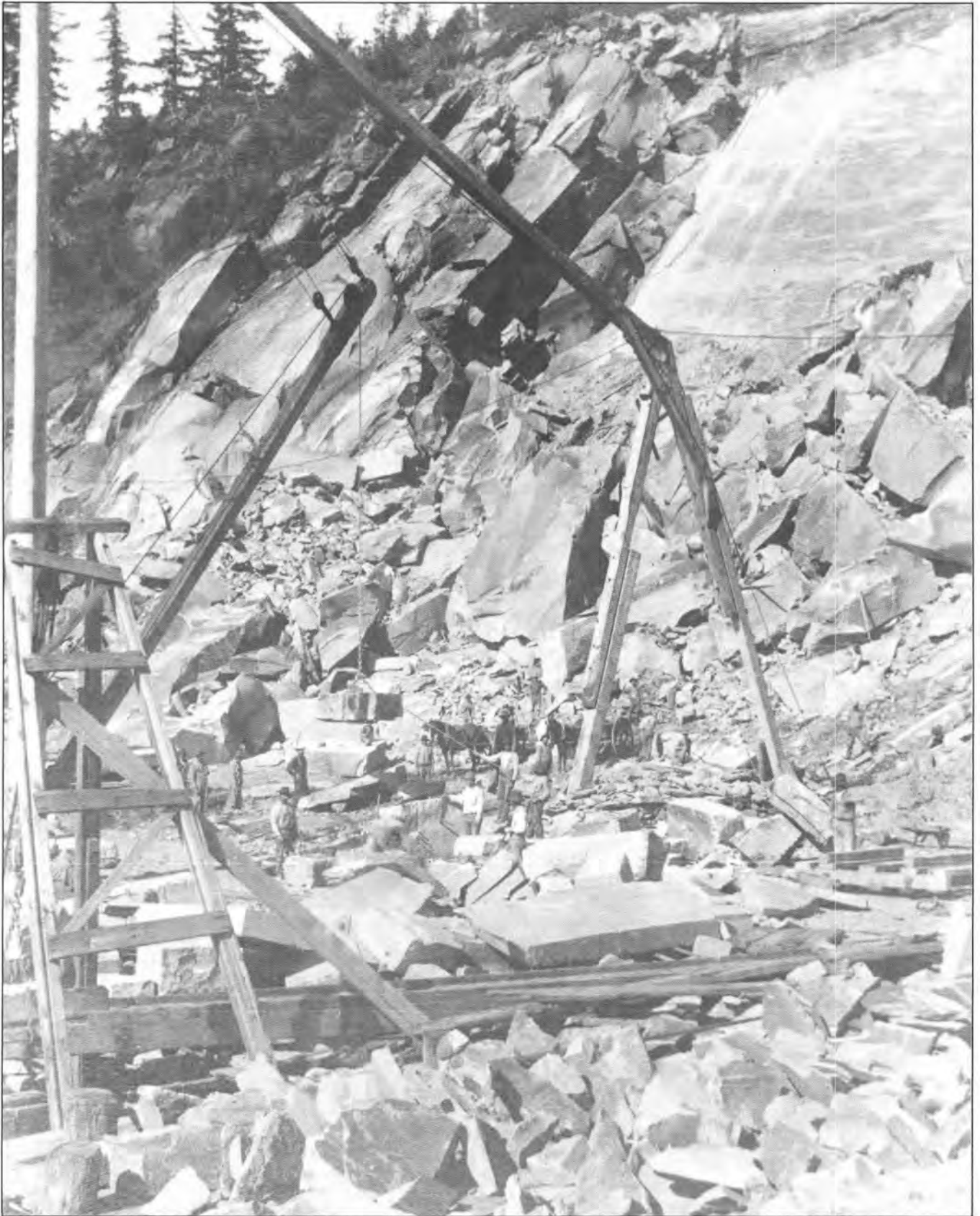
Figure 3. The Chuckanut quarry on Chuckanut Bay near Bellingham (photo taken before 1904). These irregular boulders were blasted from the steeply dipping rock face. Horse-drawn heavy-duty wagons move rock and debris in the quarry. The wooden brace on the right is a stiff-legged derrick (note size of wooden beams); this brace and guy wires (not visible here) stabilize the mast and boom on the left. The boom lifts a sandstone block encircled by a chain; steel links were typically 0.75 inches thick and chains were sectioned into 20-foot lengths. Two men on the left of the block are carrying another chain. To the right of (behind) the stiff-legged derrick, men on the rockfall are drilling holes by hand for later splitting with wedges. Typically, one person held the bit and rotated it while another person hammered; debris in the chiseled hole was removed with long-handled spoons. Photo courtesy of Galen Biery.
