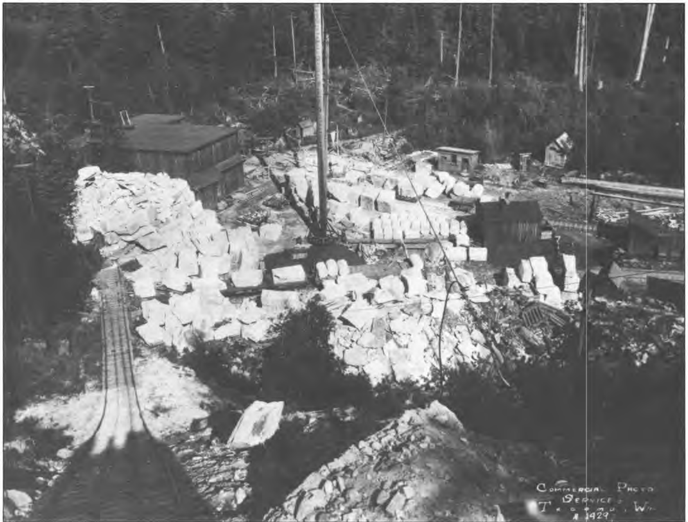
Figure 11. Sandstone at the Walker-Wilkeson quarry rough-cut as columns for the state capitol building is lying near the mast and boom derrick. These segments were shipped to the Tacoma plant and finished on a lathe. Some stones are on railroad cars awaiting shipment. The blocks of rock were let down the tramway (rails, lower left) to the saw shed. Other buildings here housed a blacksmith shop, gang saws, steam donkeys, and equipment. Photo (ca. 1926) courtesy of the Tacoma Public Library.
