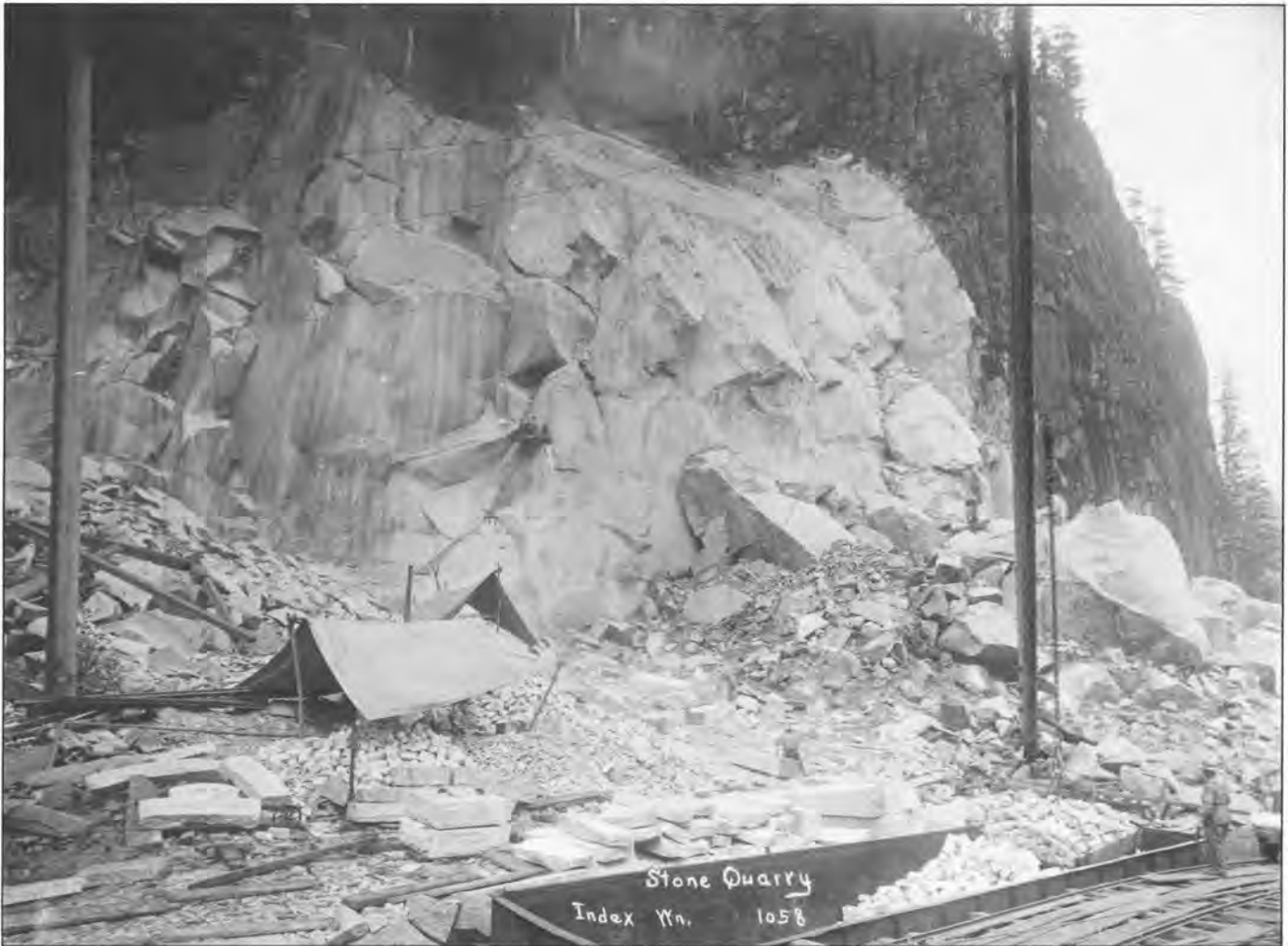
Figure 2. Western Granite Works (Soderberg quarry) at Index (date unknown). Wooden planks on two metal rods protruding from bedrock support three men who are drilling holes for blasting (center of rockface). Cobblestones were made in the tarpaulin “tents” and loaded on railroad cars for transport. The rectangular slabs behind the railroad car were split to size from irregular quarry rock and used for steps on buildings. The quarry site currently is a popular destination for technical rock climbers. Photo courtesy of Special Collections Division, Univ. of Washington Libraries, Pickett photo #1058.
