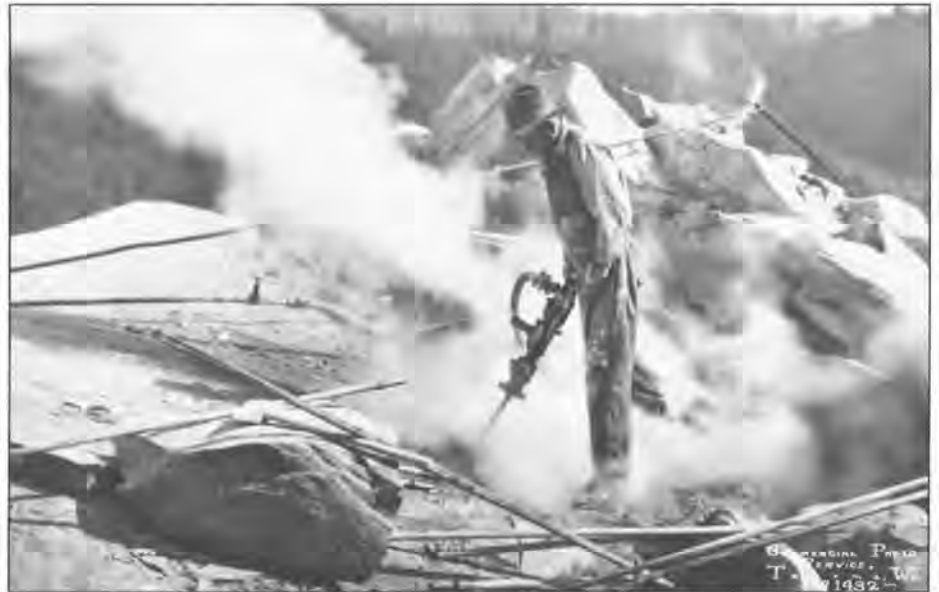
Figure 12. A drill that was converted to steam being used at the Walker-Wilkeson quarry. Rods in the foreground are drill extensions; behind the driller are steam pipes and hoses. Steam cleared the holes of rock debris. Photo (ca. 1926) courtesy of the Tacoma Public Library.
