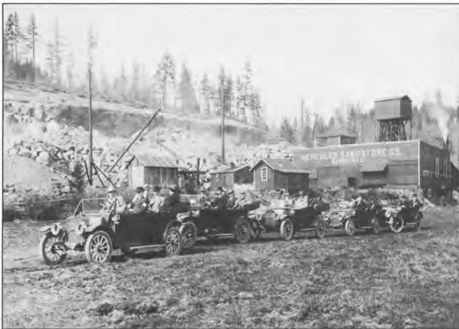
Figure 5. The day of the Big Blast at the Hercules No. 2 quarry in Tenino sandstone (Feb. 17, 1912). Stone went to the Grays Harbor jetty. People standing at the top of outcrop (upper left in this photo) suggest the scale. Projectiles from the blast put holes up to ten feet in diameter in the walls of the quarry buildings. Photo courtesy of Larry Scheel.
