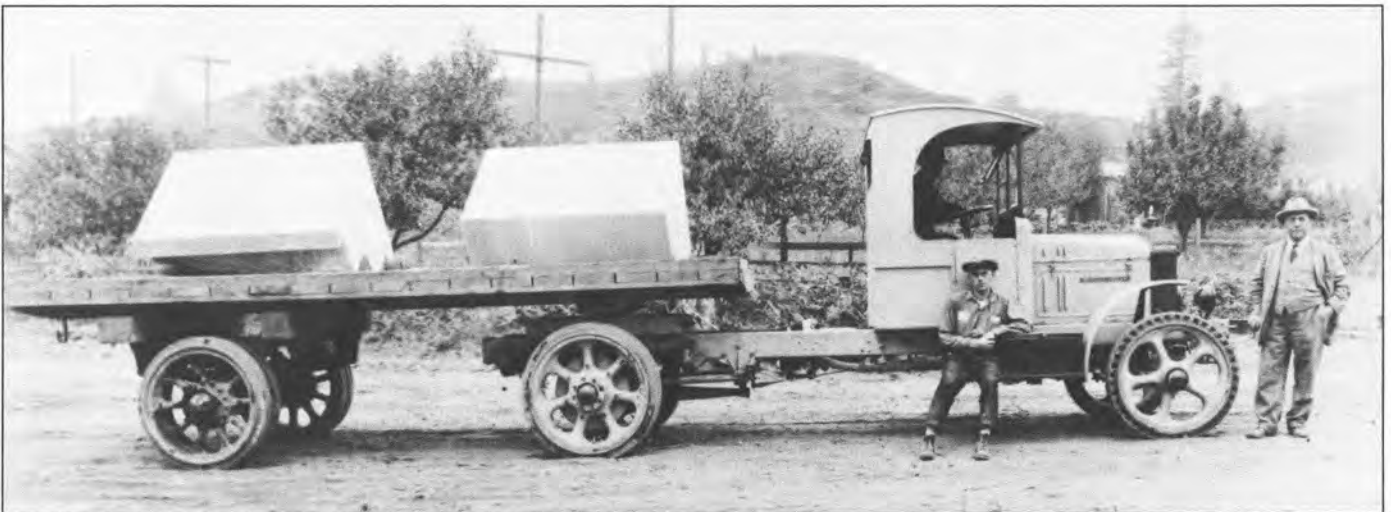
Figure 10. A GMC truck with solid rubber tires ready to haul a load of stone for the State Capitol project. The man on the right is Robert Walker, company owner. This photo was taken in about 1920 at the Center Street, Tacoma, shop of the Walker Cut Stone Company. Photo courtesy of the Tacoma Public Library.
