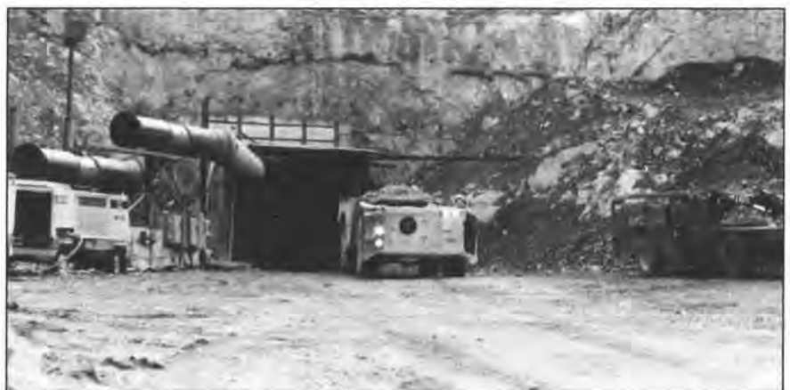
Figure 10. This adit was collared and driven 2,000 feet in 1992 to reach ore of the Lamfoot deposit northeast of Republic. The first mineralization encountered arrived at the surface in late October. The purpose of the adit was to confirm drill-indicated ore reserves: if ore reserves prove out, the adit will be converted to a full production adit in 1994. Seventy-five percent of all ore is above the level of this adit. Ore from below the adit level will be mined by ramping down to the level of the ore.
