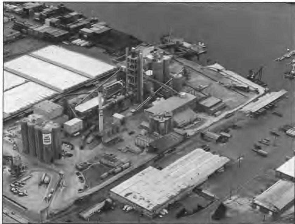
Figure 13. Ash Grove Cement Co., Western Region's 750,000 ton per year portland cement plant, located on the Duwamish River in Seattle. The plant operated for decades at this site and began producing again in May 1992 after a 5-year hiatus during which portions of the plant were either upgraded (finish grinding circuits) or demolished and totally rebuilt (clinkering plant/kilns). With its higher production capacity, the new facility is the largest dry-process portland cement plant in the northwestern U.S.
