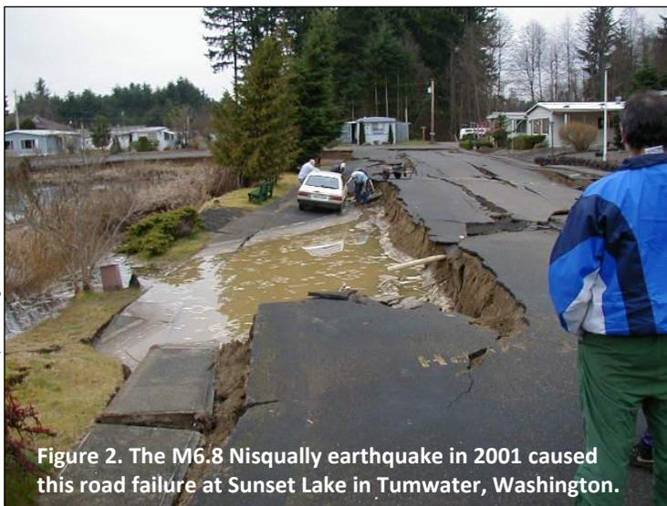
Figure 2. The M6.8 Nisqually earthquake in 2001 caused this road failure at Sunset Lake in Tumwater, Washington.
