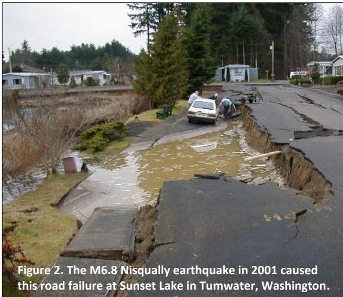
Figure 2. The M6.8 Nisqually earthquake in 2001 caused this road failure at Sunset Lake in Tumwater, Washington.
