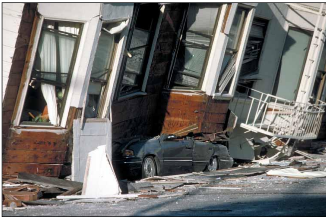
Figure 2. Sinking and collapse of a building as a result of liquefaction during the 1989 Loma Prieta earthquake in San Francisco, California. (Photo: J.K. Nakata/USGS)
