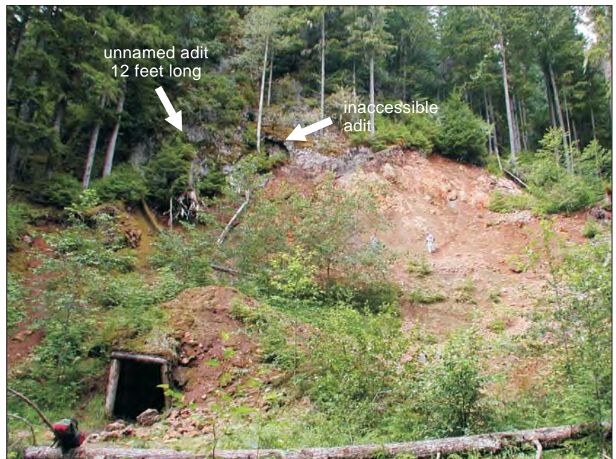
Figure 6. Portal of Mill Level tunnel in foreground and two adits in cliff; trail at far left side of photo. View to the west.
