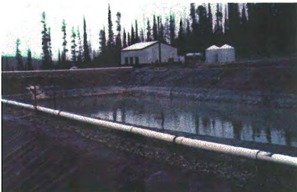
Figure 7. Pregnant solution pond during operation at the Coeur Thunder mine in 1985. Posts in foreground are about 5 feet high. (Photo courtesy of Bruce Schuld, Idaho Department of Environmental Quality.)
