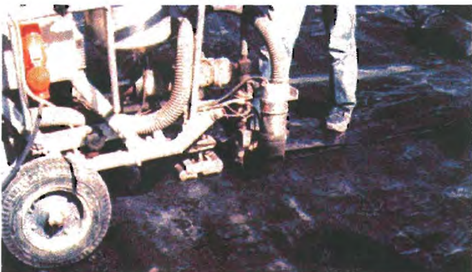
Figure 13. Installing liner systems and welding seams to prevent leaks, circa 1985. Seams have been one of the weak links in the liner process and have been a source of leaks at many sites. Improvements in welding seams have reduced the number of seam failures. (Photo courtesy of Bruce Schuld, Idaho Department of Environmental Quality.)
