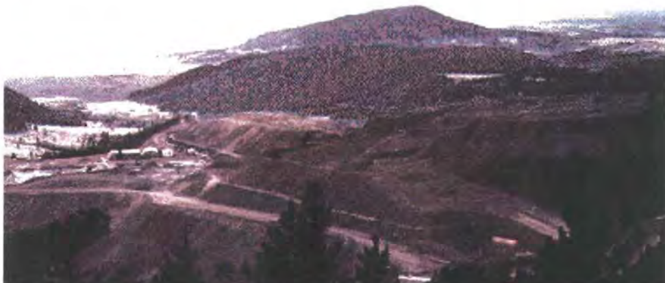
Figure 11. The Zortman-Landusky mine in northern Montana was the first to use the valley fill method. Ore is layered in approximately 30-foot lifts. Cold weather at the site requires that pipes delivering the cyanide solutions be buried beneath ore layers. Ore is not crushed at this mine, simply reduced in size by blasting and loaded on the pad. (Photo by Bob Derkey, Washington Department of Natural Resources.)
