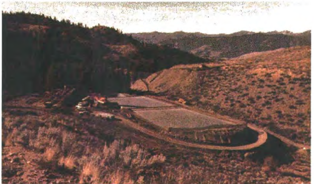
Figure 15b. Heap-leach pad at the Minnie mine prior to the placement of ore heaps. Pad liners consisted of single layer geomembrane placed on a compacted soil base. Pads are 120 ft x 120 ft. (Photo by Rod Lentz, U.S. Forest Service, Okanogan National Forest.)
