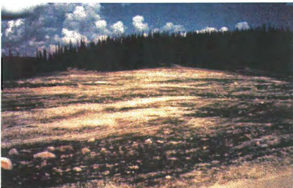
Figure 8. Reclaimed heap-leach pad in 1993 at the Coeur Thunder mine, approximately 2 years after mining was completed. Spent ore was unloaded from pads and placed in mined-out pits. Photo shows approximately the same location as that in Figure 6. The recent drought has limited growth at this site. However, grass and pine trees have begun to spread as conditions become more favorable.
