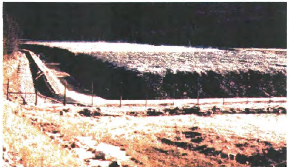
Figure 4. Heap-leach pads at Minven's Stibnite mine in central Idaho. Fence posts in foreground are about 6 feet high. Sprinklers apply cyanide solution to the ore. After trickling through the heap, solutions are collected in ditches at the perimeter of the heap and directed toward the pregnant solution pond. (Photo by Allen Throop, Oregon Department of Geology and Mineral Industries.)
