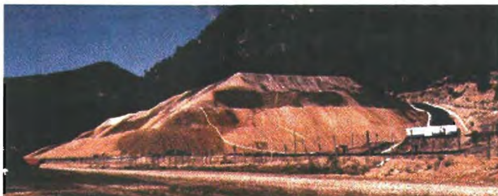
Figure 9. Hecla Mining Company's Yellow Pine, Idaho, heap-leach facility. Lifts are approximately 20 feet high, resulting in an 80-foot high heap. After each layer of the heap is leached, a new layer is placed on top and leaching continues.
