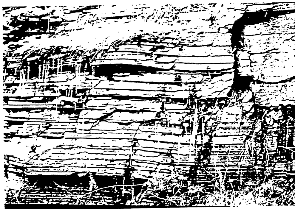
2 D (with minor, irrelevant vertical cracks)
