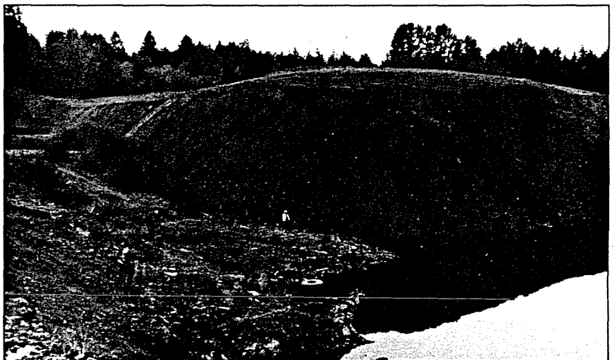
Figure 6. In the top photo, overburden is stacked on top of a highwall left by mining, ready to be bulldozed into position. The short push will reduce the cost of reclamation. In the bottom photo, moving of overburden into position for reclamation is nearly complete. Overburden has been pushed over the highwall with a bulldozer. Blast casting was attempted here to reduce costs; however, the shot holes could not be kept open because the overburden is unconsolidated. The final reclaimed slopes allow easy escape from the pond and will be revegetated. Lower photo by M. A. Shawver.
