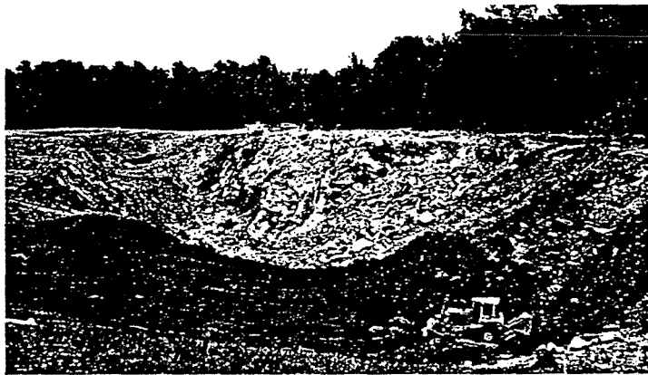
AFTER: In September 1990, the pit had been virtually reclaimed except for two remaining highwall shots in center of photo.
