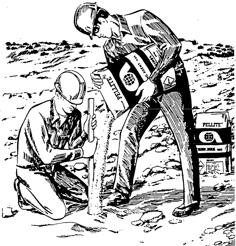
Figure 3-6. AN-FO mix packaged in 50-lb bags. (Reprinted from Atlas Powder Company, 1987, Explosives and Rock Blasting , figure 5.3.)
