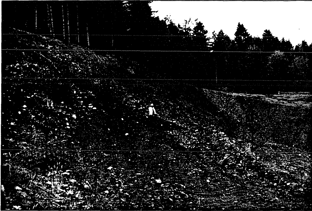
Figure 7. This slope was backfilled using material from the site. Additional material needed could not be taken from adjacent land because it was not part of the permit area. The expense of hauling in material made reclamation costs for this segment higher than the actual value of the rock mined. The belly scraper used to place material compacted the slope to make landsliding less likely. Alder trees, which are nitrogen-fixing plants that enhance soil fertility, will be used in revegetation to complete the reclamation of this segment.
