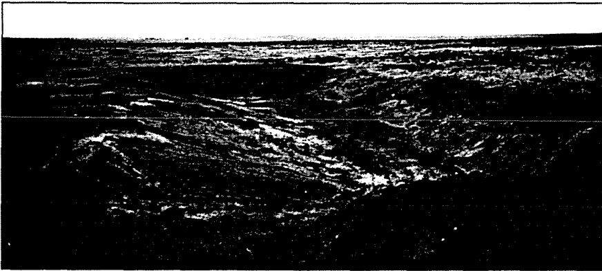
Figure 12. Slopes in this eastern Washington basalt quarry were reduced by moving unused blasted rock and overburden from around the edges of the pit, which is approximately 150 feet by 400 feet. Revegetation has occurred only in areas where soil was present. Photo by Clint Bigger, Adams County Public Works Department.
