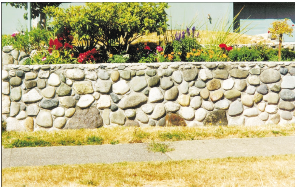
Figure 1. A mortared stone wall in western Washington. Notice that it is thinner and more vertical than the wall in Figure 2. Photo by Wendy Gerstel.
