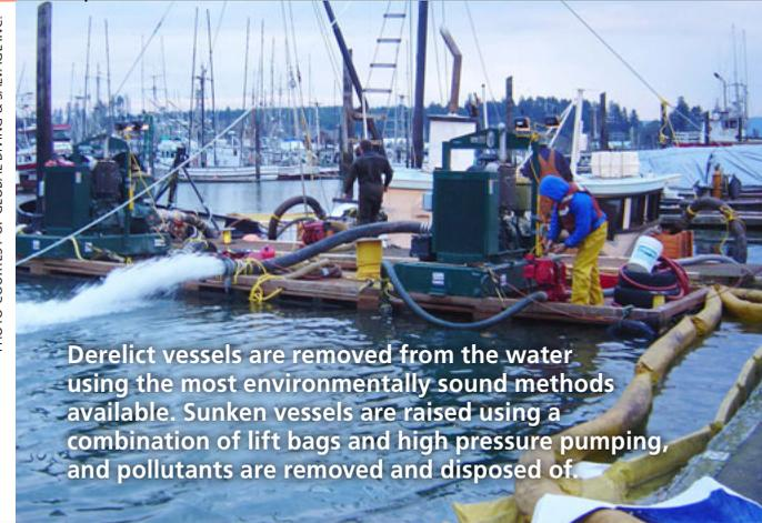
Derelict vessels are removed from the water using the most environmentally sound methods available. Sunken vessels are raised using a combination of lift bags and high pressure pumping, and pollutants are removed and disposed of.
