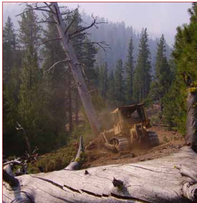
Hazard tree, too fragile for manual felling without injury can also be pushed over.
