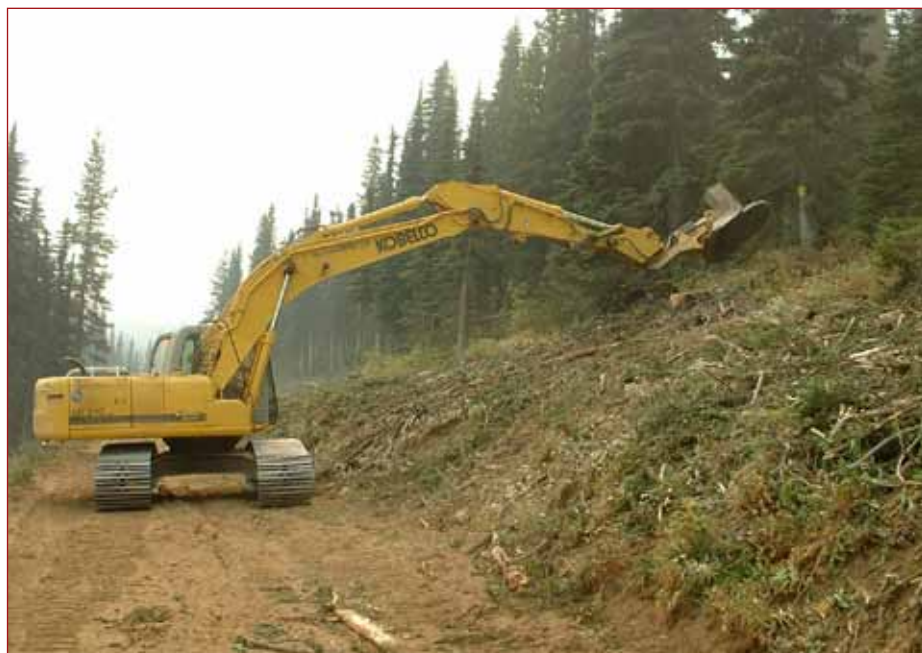
Roadside mulching to increase travel route visibility and reduce ladder fuels.
