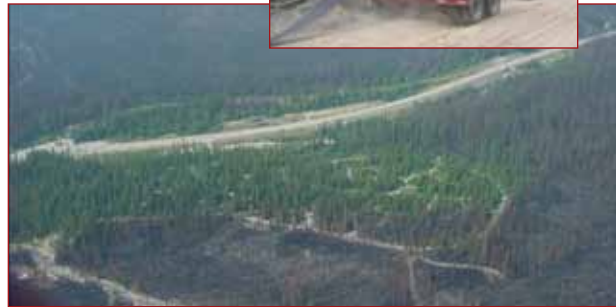
Marble Canyon Campground - Successful Protection with High Volume Sprinkler System - Kootenay Fire Complex
