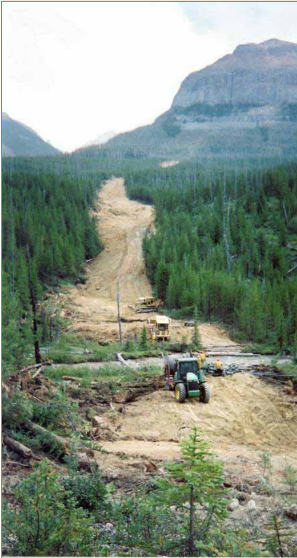
High Volume Sprinkler Protection System Setup Kootenay Complex, Vermillion Pass, Canada, 2003
