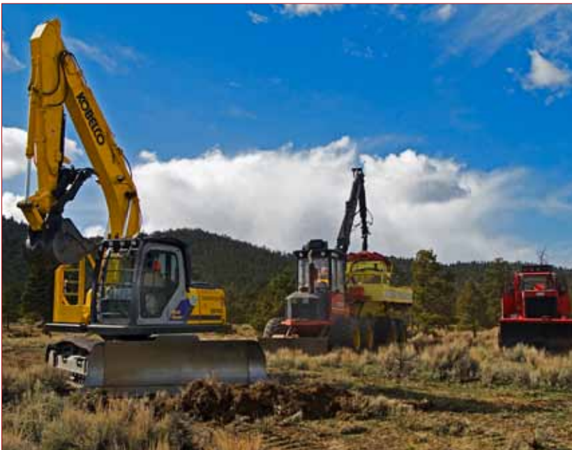
Good holding task force (excavator, super-skidgine, soft-track skidgine)
