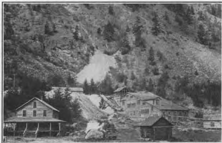
New camp buildings and concentrator at Ruby Mine.
