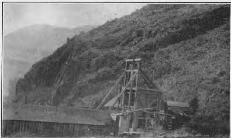
Head bin and hoist room for inclined shaft on Kaaba vein. The vein outcrops along the base of the mountain.
