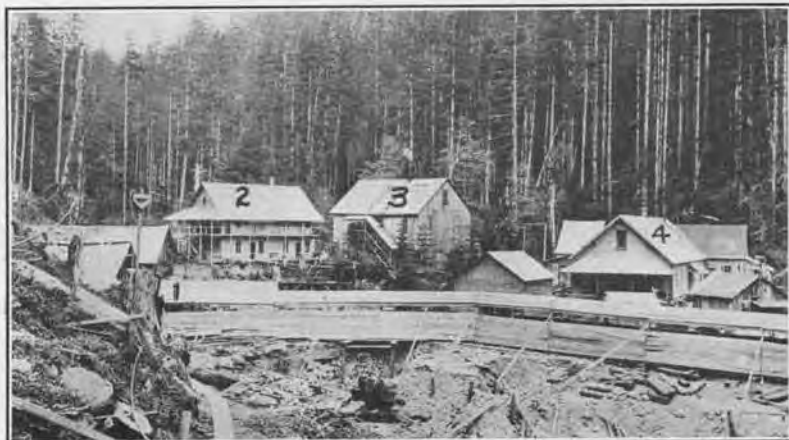
Camp of the Sunset Copper Company. (1) Portal of the main adit, (2) and (3) bunkhouses, (4) boarding house.
