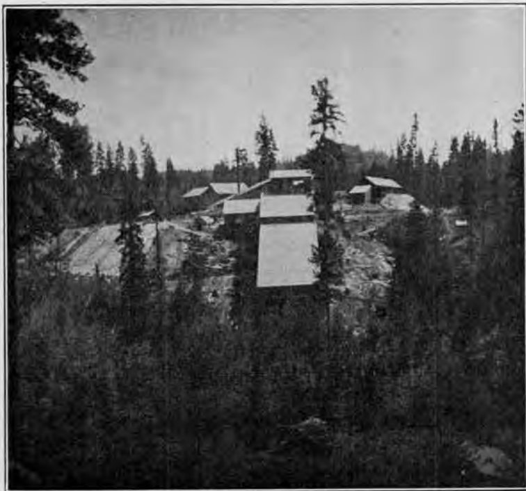
New all-flotation mill and surface plant of the Loon Lake Copper Mine.
