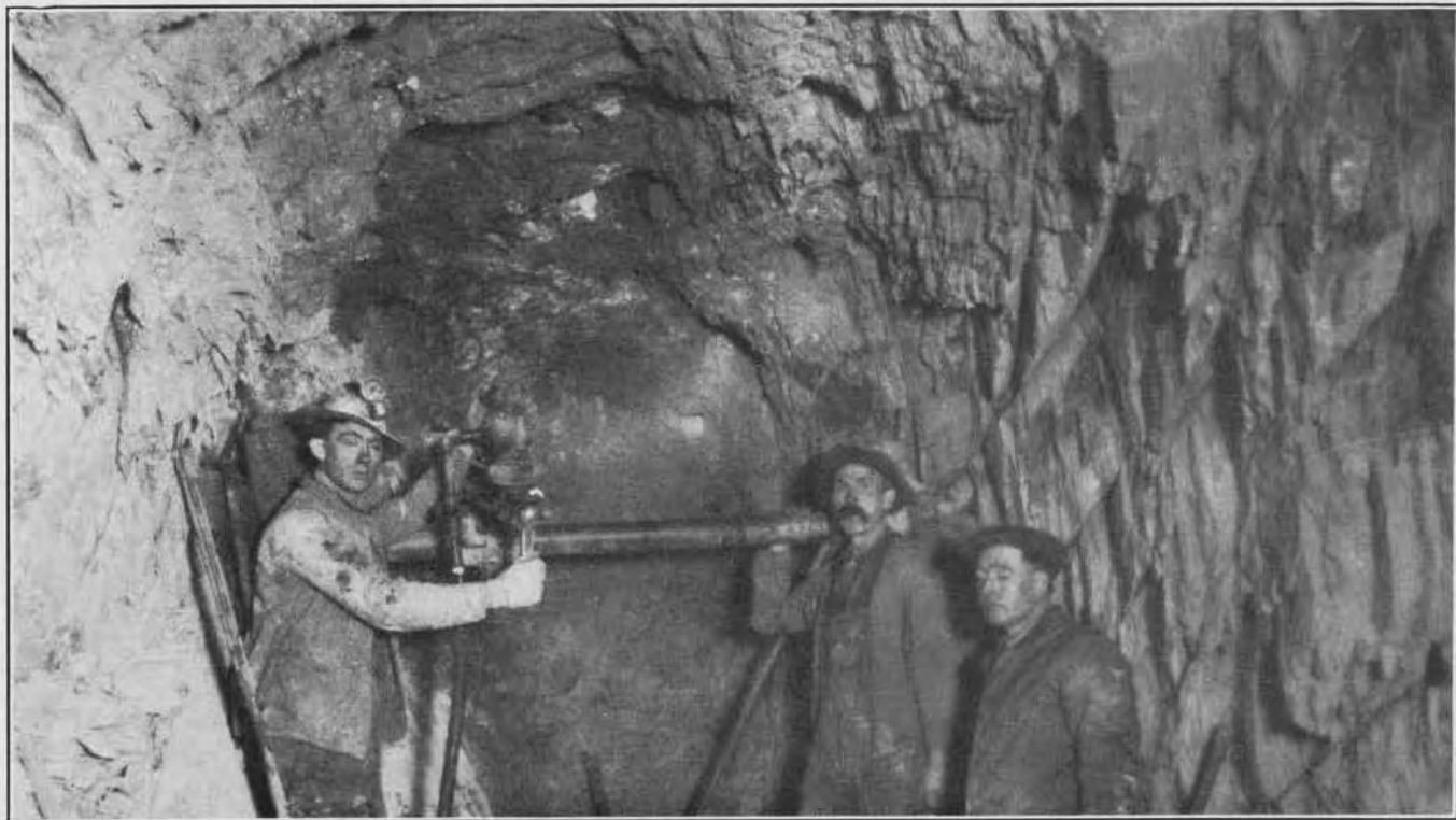
Drifting on the United Copper Vein, 1200-foot level.
