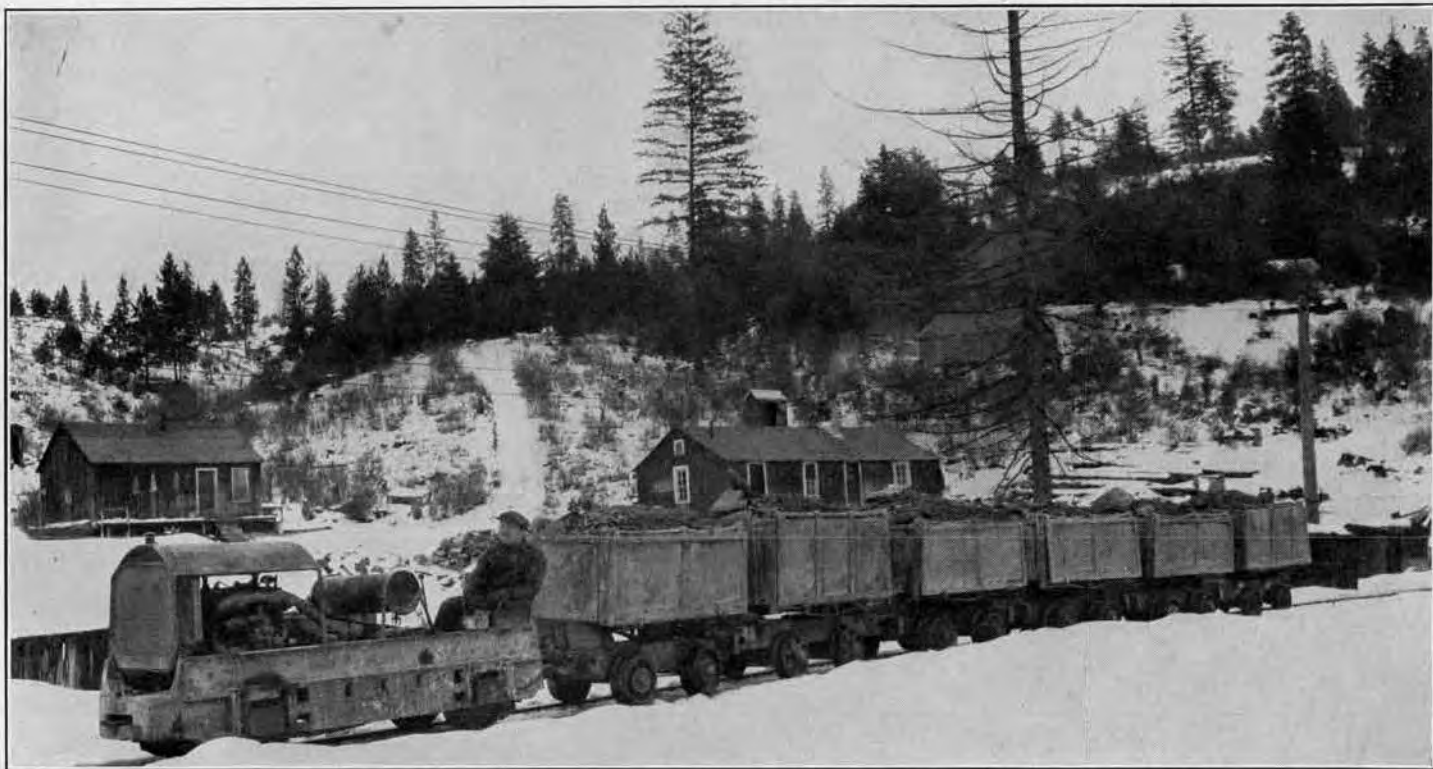
Gasoline locomotive hauling train of ore from main adit of United Copper Mine.
