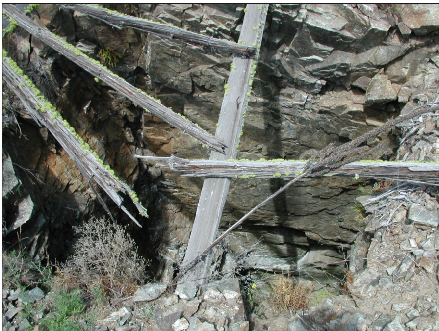
Figure 15. Upper photo shows one of several open shafts on Palmer Mountain with a collapsed fence around shaft opening. Loose rock around the shaft collar increases hazard. Lower photo shows view down shaft.
