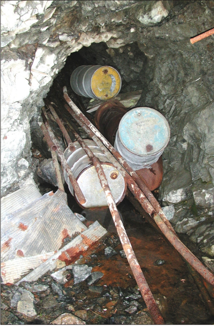
Figure 6. Discarded barrels, piping, and sheet metal in adit at Florence Rae mine.
