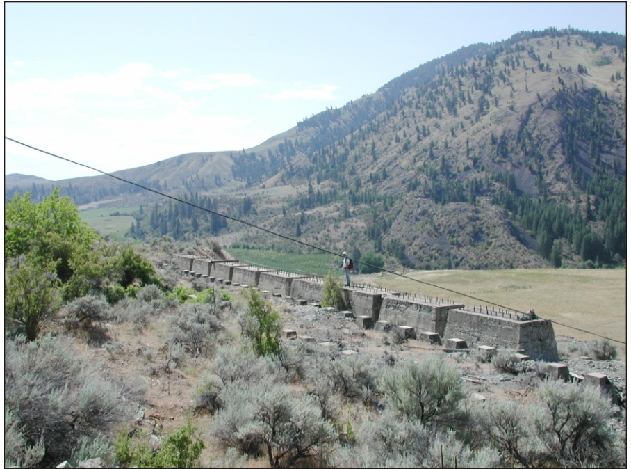
Figure 11. Concrete foundations for the nine-stamp mill at the base of Palmer Mountain. Foreground and background show the open, sparsely vegetated geography of the Cecile Creek WAU. View to the southwest.
