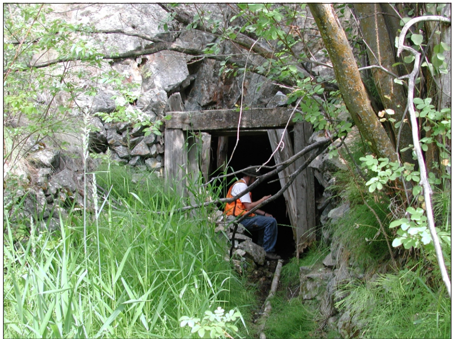
Figure 14. Lower adit at the Security mine. Drainage from the adit forms a small oasis in otherwise dry shrub-steppe environment. Water samples revealed no significant water quality problems. Cool air flowing from adit indicates possible bat habitat.
