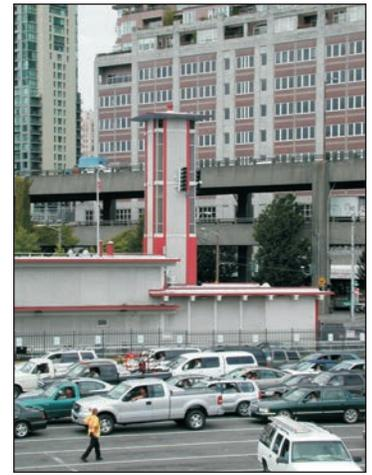
**Figure 8.** The AHAB radio warning system tower (red trim) at Colman Dock ferry terminal on the Seattle waterfront. Seattle AHAB stations use seismic instruments, cameras, a weather station, and chemical sensors to detect natural and man-made hazards. They can also be activated by NOAA Weather Radio. A siren and a loud voice message tell the public how to seek safety. View to the north.
