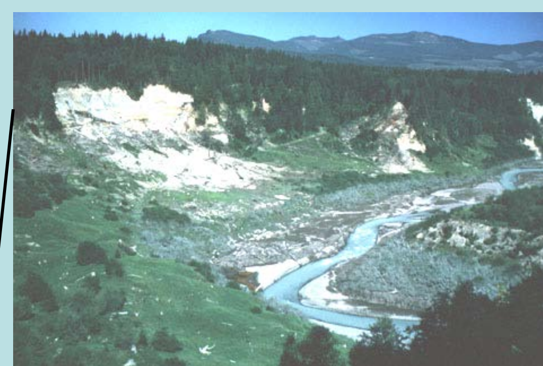
Landsliding upstream of the Mud Mountain Dam along the White River. Failures occur due to geologic materials that are constantly being wetted and de-watered during winter water retention periods of high stream flow.
