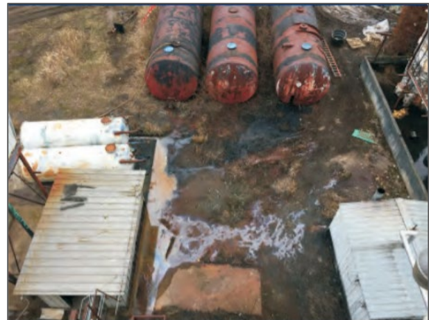
Figure 15. Impacted soil at Treoil site during EPA cleanup (Photo: Valeriy Bizyayev, 2017).
