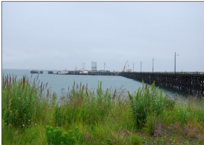
Figure 20. Phillips 66 Pier. (DNR photo).
