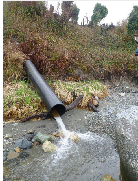
Figure 5. Image of stormwater runoff onto the beach in Birch Bay (DNR 04/08/2014).
