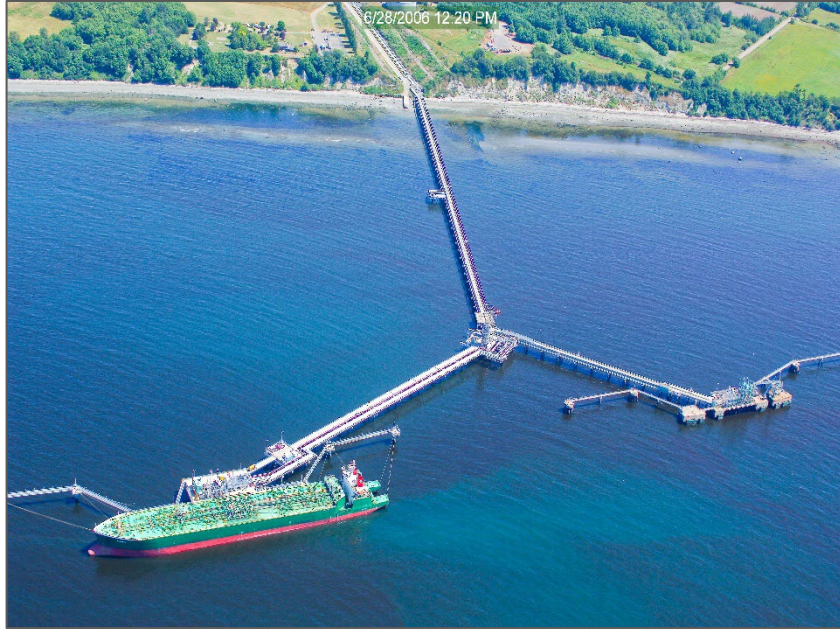
Figure 18. bp Pier ( Ecology Coastal Atlas ).
