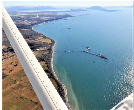
Figure 17. Aerial view of Cherry Point piers (Photo: Christopher Krembs, Eyes Over Puget Sound, WA Ecology).
