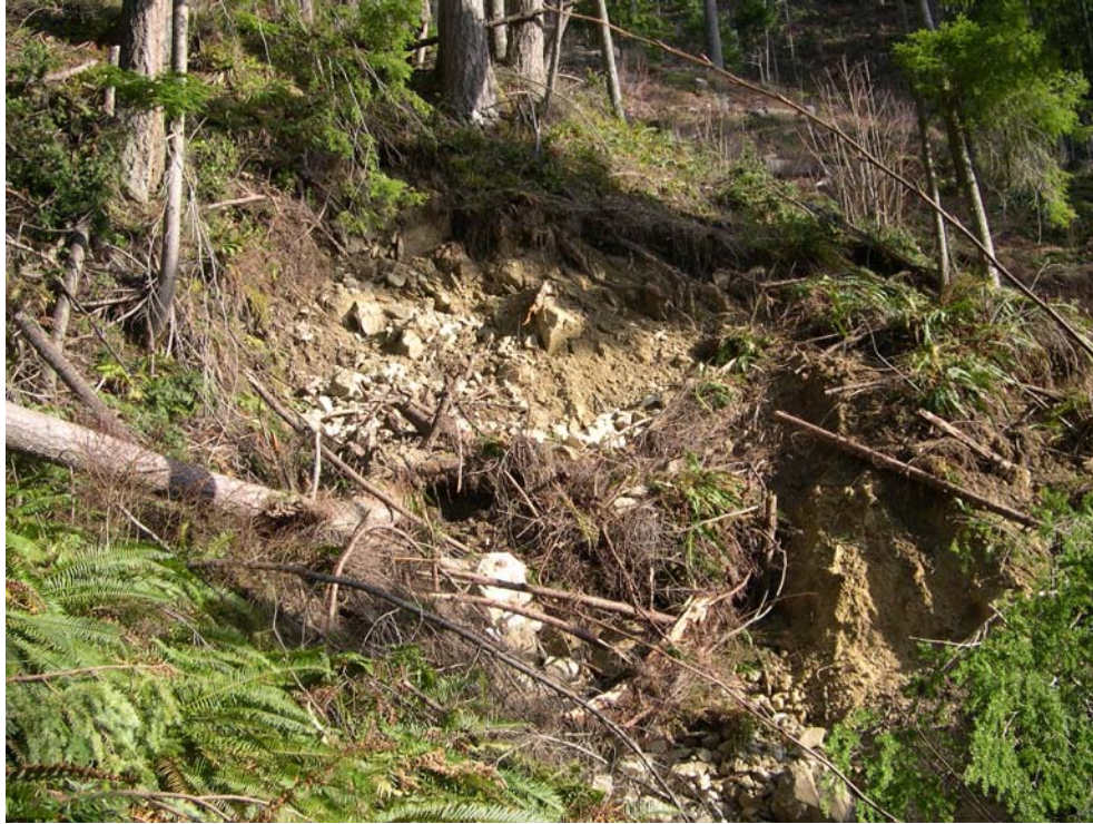
Figure 8. Way South #1 PI Scar. View looking south. (Photo by Casey Hanell, 2009)
