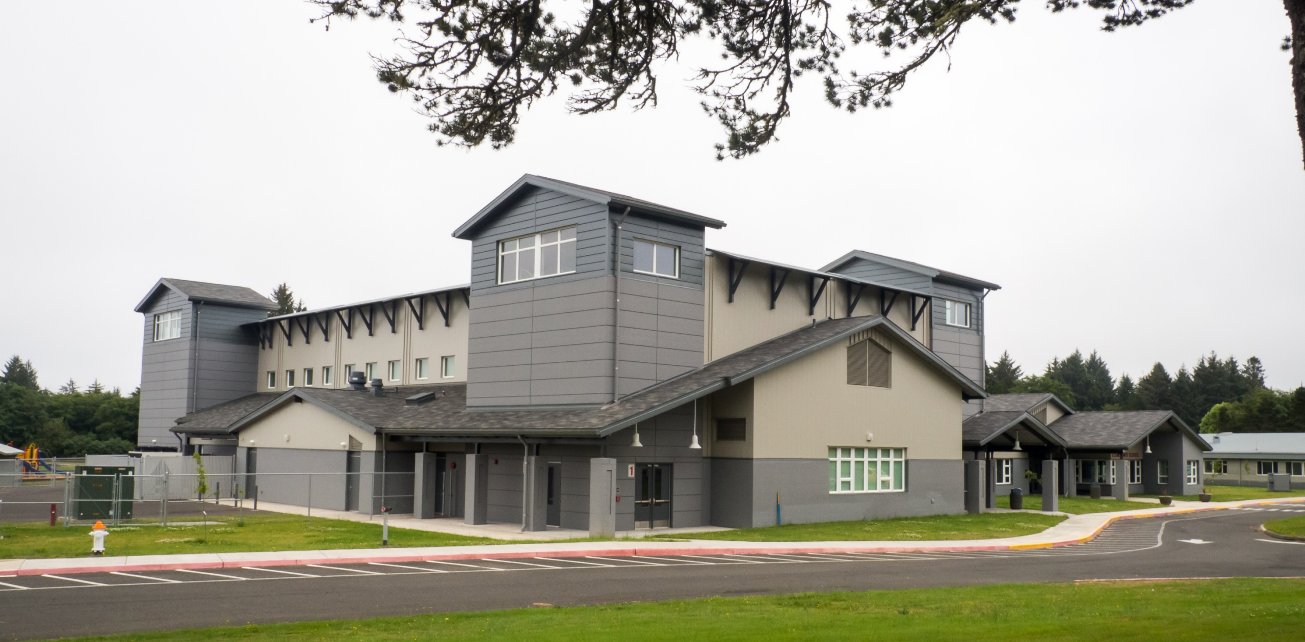
Ocosta School vertical evacuation structure
