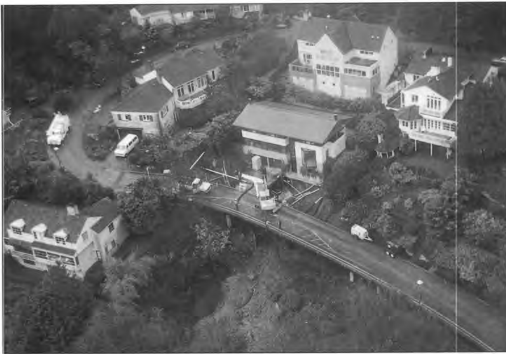
Figure 2. This house, which has been the subject of several news stories, is located on East Boston Terrace in the Capitol Hill area of Seattle. It hangs precariously over the headscarp of a reactivated old landslide. Careful construction engineering preserved the structure but not the front yard, leaving the driveway suspended. The failure of the front yard destroyed part of the road below. Note the exposed pipes, climbing ivy no longer rooted (below the tall window on the right), and tension cracks migrating into the neighbor's yard to the left in the photo. After this picture was taken, a retaining wall was built in front of the house (Seattle P-I, Feb. 6, 1997); a retaining wall behind the house was built during the original construction. This house is in the same drainage as, and a few hundred feet upslope of, a house destroyed by a landslide in 1942. That landslide killed one resident and seriously injured another.
