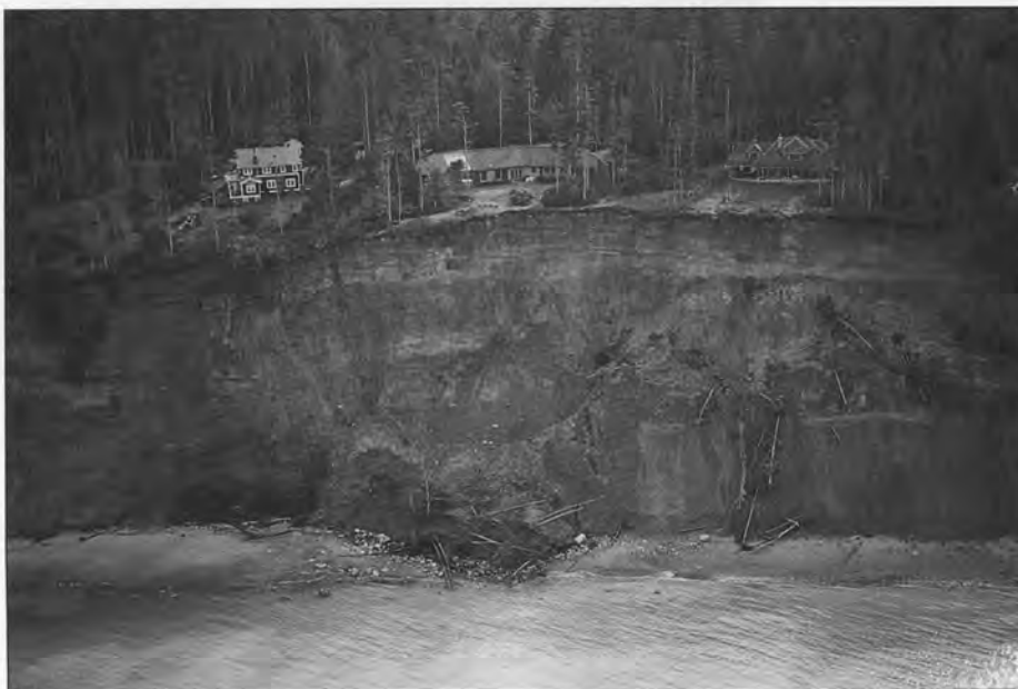
Figure 17. Fortunately, homes here were built with adequate setback—for these failures. The depth of a failure surface can influence the rate of retreat of the edge of the upland surface. In this slide west of Port Townsend, shallow debris avalanching (far left) has caused no significant edge retreat yet. The mid-bluff bench on the right indicates a relatively deep-seated slide of upper-bluff sediments only. (See Fig. 21B.) The surface of failure for the middle slide is even deeper, "daylighting" at (or below?) beach level (Fig. 21B, C), and has caused the most retreat. At many sites along the coastal bluffs, sedimentary units are not laterally continuous, and conditions can be quite different over a distance of 100 feet or less.
