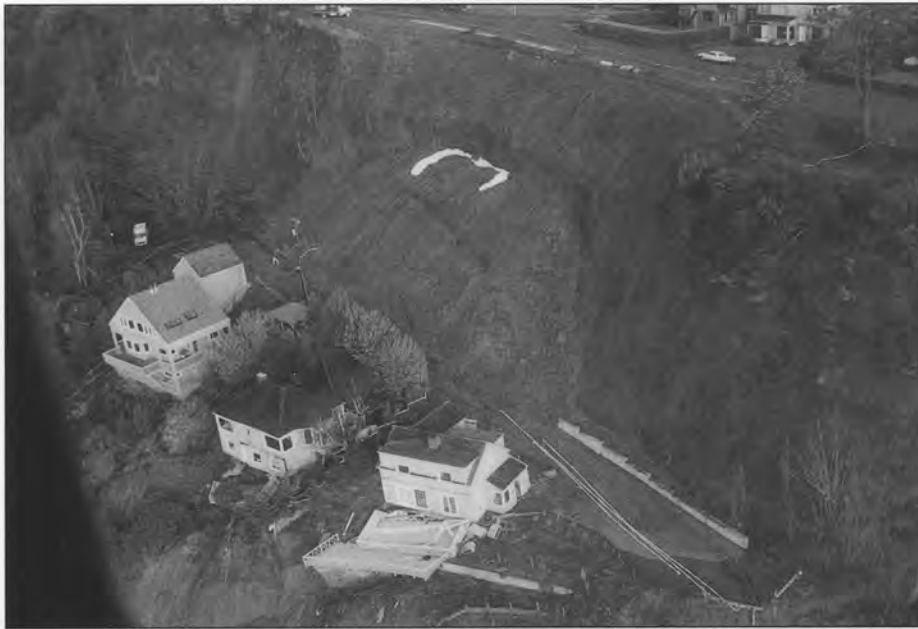
Figure 6. This photo shows one of the larger landslides along Perkins Lane on the southwest side of the Magnolia neighborhood. This is an area of continuing large-scale instability. Immediately following the February 1996 storms, a 1,500-yd 3 landslide (Harp and others, 1997) slid from the upper portion of the bluff into the back yard of the home on the right. Seattle engineers attempted to mitigate the problem by regrading and revegetating the upper slope. However, the February landslide was a shallow manifestation of a deep-seated rotational failure that formed, or might have already existed, in the sand, gravel, and silt deposits of the bluff at this site. This deep-seated slide was reactivated in December 1996, damaging at least five houses. These three are now uninhabitable. The white plastic sheeting on the slope was probably placed there in an attempt to prevent water from infiltrating the soil. This site is representative of the geologic conditions shown in Figures 20 and 21C.
