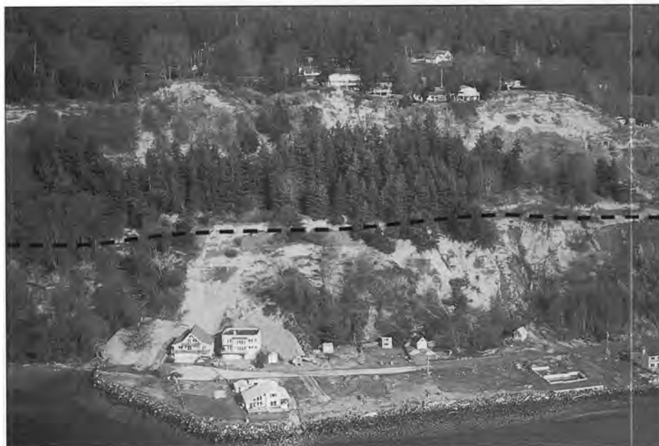
Figure 14. At Scatchet Head at the southern end of Whidbey Island, mudflows temporarily block access to these beach-level homes during wet winters. The upper bluff is porous glacial outwash sand that dries out in summer. The silt that forms the lower bluff (below dashed line) and perches ground water is damp and green year round. The top of the silt is approximately at the position of the dashed line. The scarp in the background and the partially forested bench are characteristic of such slide areas where percolating ground water is perched above the less permeable silts. The sands are weaker than the silts and slide readily when saturated. Similar situations are present north of Carkeek Park and in the Golden Gardens area of Seattle, among other places. (See Figs. 20, 21.)
