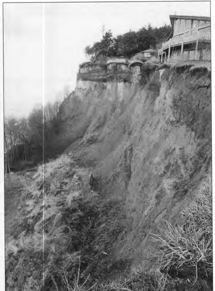
Figures 19A & B. Continuing slide activity has made this home near Cape George in Jefferson County uninhabitable. At this site, the perching layer is a small area of ancient lakebed silt that lies beneath the house at about mid-bluff level, now covered with grass dropped from the back lawn. This part of the bluff remains green year round. Note the old slide mass at beach level (lower left), now covered by alder trees that are all of approximately the same age (here, perhaps 25 years old). Also note the arcuate line of boulders seaward of these trees. Such a pattern of boulders, which are commonly accompanied by steeply tilted silt and clay beds, can indicate an old slide surface at or below beach level. B. (right) This closeup shows recent slide debris on the bench, as well as the exposed septic tank (the white rectangle below the right side of the house and drainfield pipe in A); the tank has since fallen to the beach. Poorly located septic systems often contribute to slope instability. The dark strata at the upper part of the bluff are gravels and are not saturated here. It is possible that drainfield effluent percolated downward and bluffward to destabilize this slope or that deeper ground water caused the problem at this location. Wave erosion has likely been a contributor at this site as well. Trying to maximize a view by building close to the bluff line can be a costly and potentially hazardous mistake.
