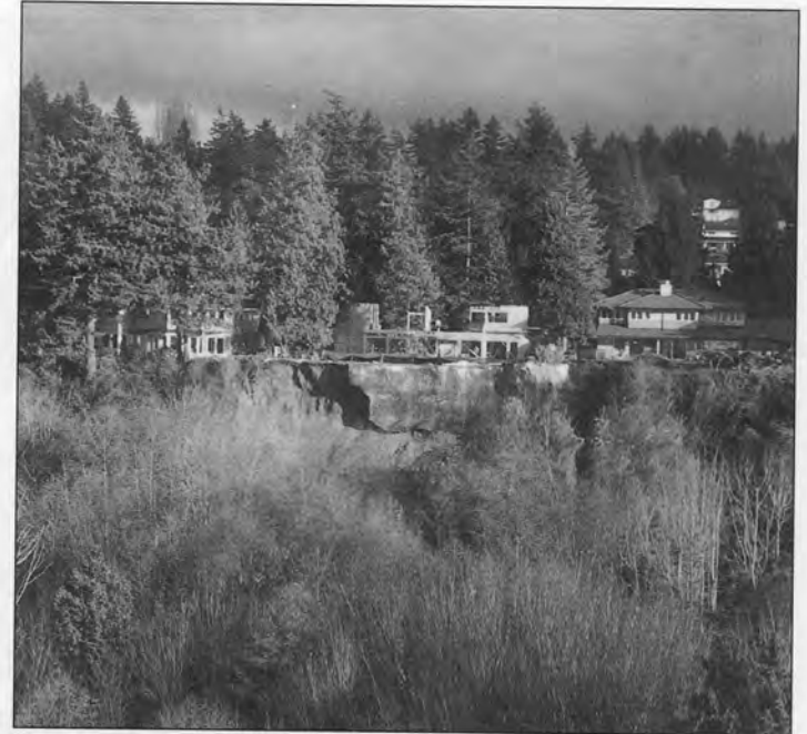
Figure 11. The owners of the house under construction in the center of this photo recognized the potential for instability at the site. The "shotcrete" (concrete sprayed on the slope) on the face of the slope was intended to protect the sandy upper part of the slope from surface erosion, but failed, probably due to excessive hydrostatic pressure. The shotcrete seems to hang like a curtain over the bluff face, with the left portion having fallen away.
