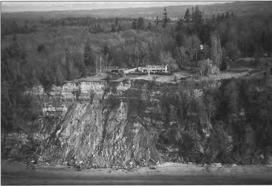
Figure 15. Slide activity such as this in the Useless Bay area of Whidbey Island can cause periodic retreat of the bluff edge by as much as 20 feet or so in seconds. During this recent slide, a portion of the fence in front of the large house was lost. Such episodes commonly are preceded and followed by decades of little erosion, making estimates of average bluff retreat rates potentially meaningless. In this location there are multiple impermeable silt layers that perch water, in contrast to conditions like those at Scatchet Head (Fig. 14), where water is concentrated above one impermeable "perching" layer. Slides here can be triggered by an abundance of water (as in the December/January storms) or by wave erosion at the base of the bluff. A rainstorm may simply be the "last straw". In many locations around the sound, water from winter rains is accumulated inland of bluffs and may cause landslides to occur months later as it slowly migrates toward the bluff. In the mid-1970s in the Golden Gardens area of Seattle, slides occurred well into summer after a series of exceptionally wet winters.
