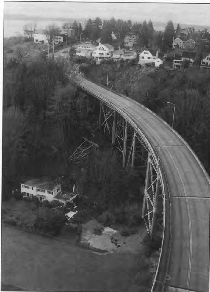
Figure 10. This view to the west over the Magnolia Bridge, a major artery into downtown Seattle, shows the landslide that forced the closure of the bridge and the "red-tagging" (condemning or declaring uninhabitable) of at least five homes along the headscarp of the slide. This slide occurred after the rains had ceased. Notice the displaced bridge trusses, the debris on the house at the base of the slope, and the broken water main just below the fallen truss and above the house.
