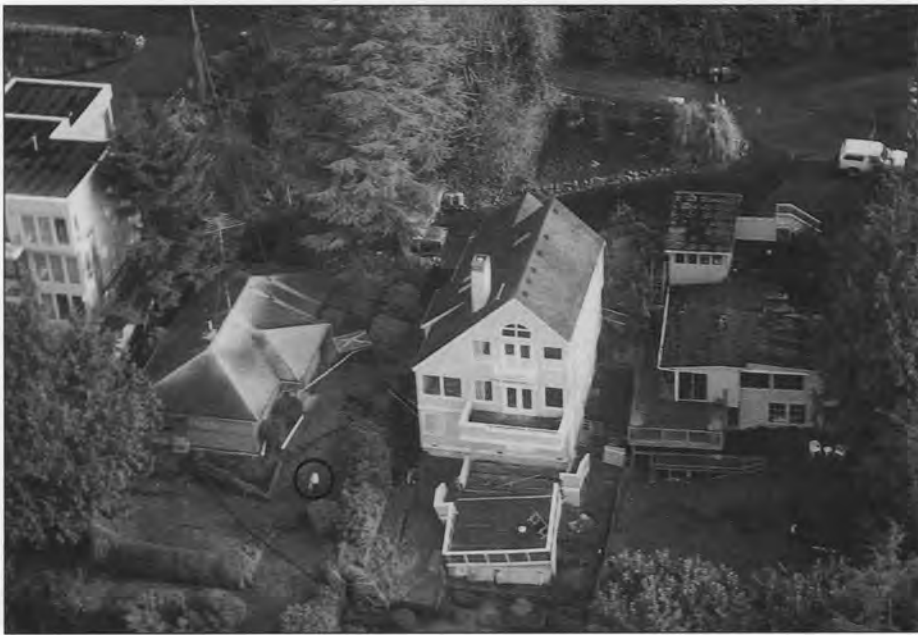
Figure 5. This view to the east shows three homes along Alki Avenue SW in West Seattle that were affected by a growing deep-seated landslide. The largest displacement occurred west (toward the viewer) of the low house on the left. Note the person (circled) standing on the down-dropped portion of the slide in front of the headscarp. Also visible is the displacement of the deck of the large house in the center. The tension crack delineating the headscarp continues through the deck area in the center house and into the backyard of the house to the right (south). The dark line extending from the house on the left is a tightline for drainage (see p. 29). Another segment of the headscarp is visible to the left of the tightline.
