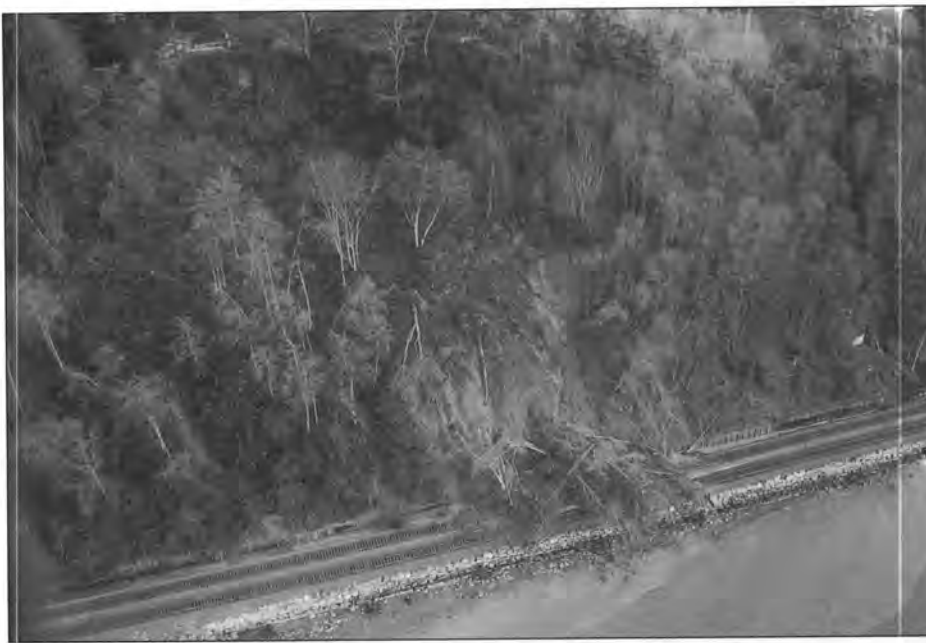
Figure 12. This slide, one of many that occurred along a stretch of railroad tracks north of Carkeek Park, lies within an older, larger slide scar. Past slides along these tracks have temporarily halted train traffic many times. Such slides have knocked railroad cars into Puget Sound, at times resulting in injuries or hazardous spills. Trip wires are strung just above the retaining wall along the tracks. An interrupted circuit signals when (but not precisely where) landslides occur. Figures 21 through 26 illustrate the different mechanisms responsible for landsliding along this stretch of bluff. Development at the top of the bluff can contribute to and is affected by the slides. Coastline modifications such as the bulkhead (built in the 1890s to support the railroad bed) also affect slope and near-shore processes. The bulkhead does not prevent landslides, but does control the rate and nature of redistribution of slide debris in the near-shore zone. Material dumped into the Sound by railroad crews cleaning the tracks is rapidly redistributed out of the narrow and steep intertidal zone and offshore by wave energy reflected off the bulkhead.
