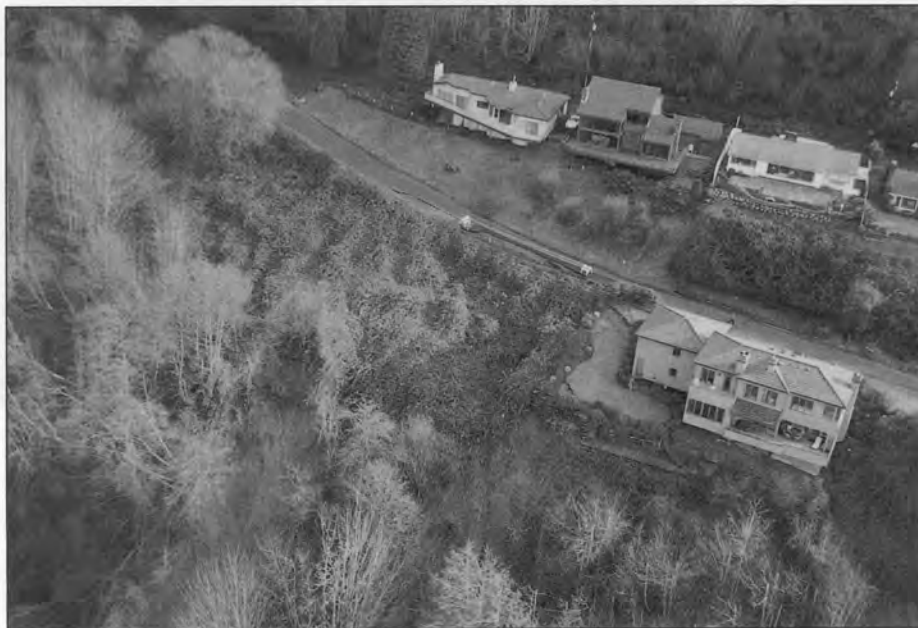
Figure 7. This house in West Seattle (lower right), and a portion of the road that runs behind it, are built on fill, commonly failure-prone when saturated. Note the down-dropped (and previously patched) section of the road between the white signs. Tension cracks start to the left of this area and extend to the right, under the house. Fill material at the lower right corner of the house appears to be displaced. Also note the recent debris flows in the drainage below the road (lower left center of this photo). These may have been caused by excessive runoff onto colluvium and fill.
