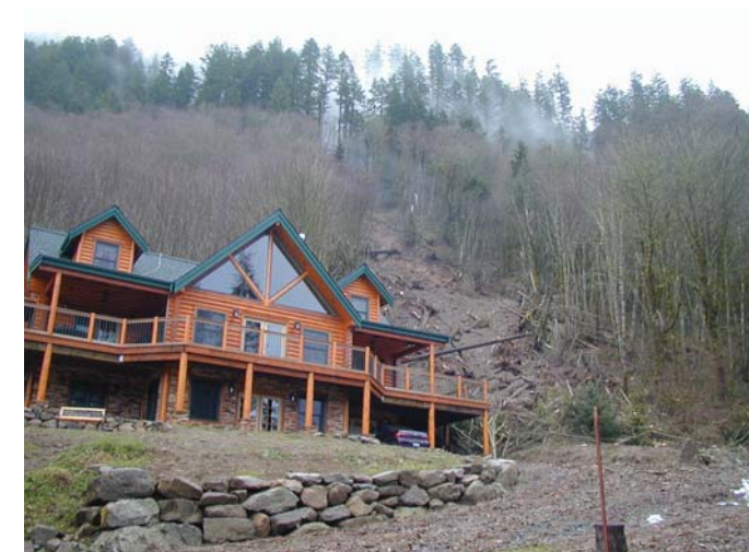
A debris flow missed this house in Whatcom County. Photo: Jeff Grizzel
