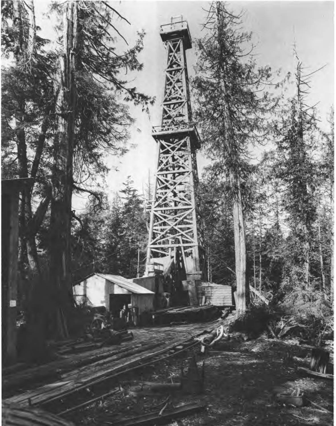
DRILLING OPERATIONS of the 1930's near Jefferson Cove where eleven oil test wells were drilled and substantial oil shows were reported (Photo courtesy of Jones Photo Shop, Aberdeen, Washington) (fig. 18).
