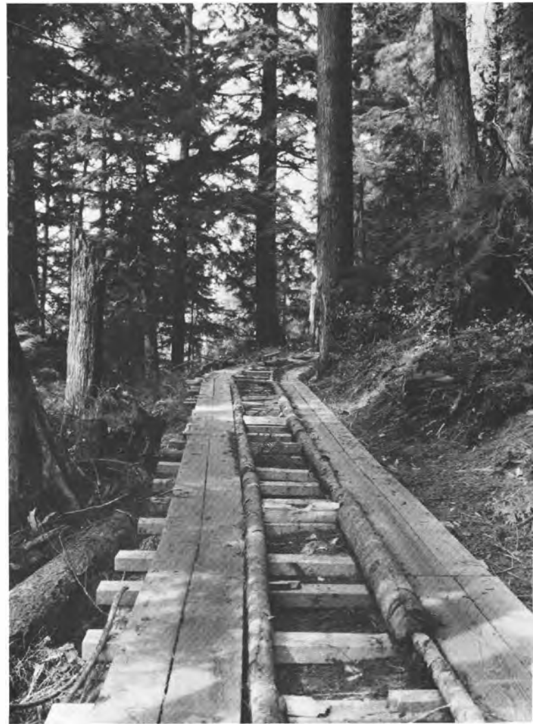
THE PLANK ROAD that served as access from the Hoh River to the Jefferson Oil Seep area as it looked in the 1930's. Barely recognizable segments of this road can still be traced (Photo courtesy of Jones Photo Shop, Aberdeen, Washington) (fig. 19).
