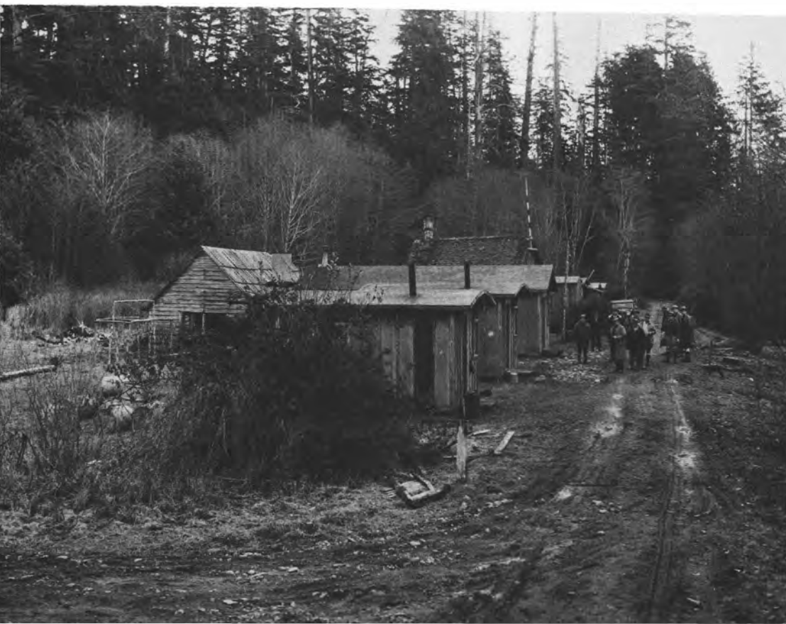
OIL CITY in the 1930's, near the mouth of the Hoh River, served as the headquarters for drilling operations at the Jefferson Oil Seep area 2 miles to the north (Photo courtesy of Jones Photo Shop, Aberdeen, Washington) (fig. 21).
