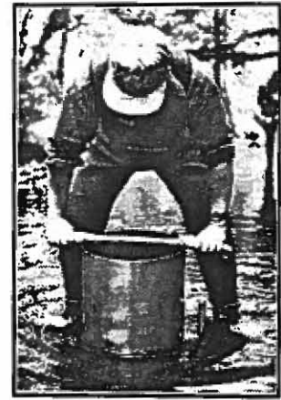
Figure 7. Forcing cylinder into gravel.
