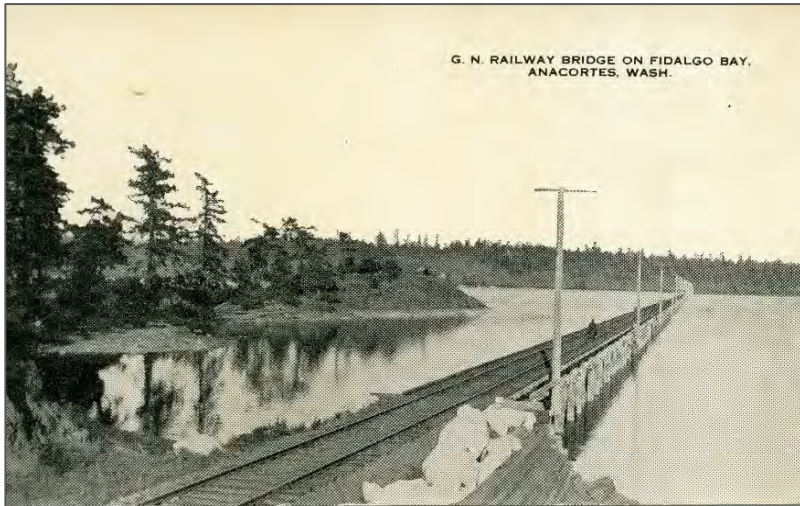
Figure 15: Photo from 1907 of railroad trestle looking east from Weaverling Spit. Note wooden piling construction of entire trestle prior to causeway construction ( Photo courtesy of Anacortes Museum ).
