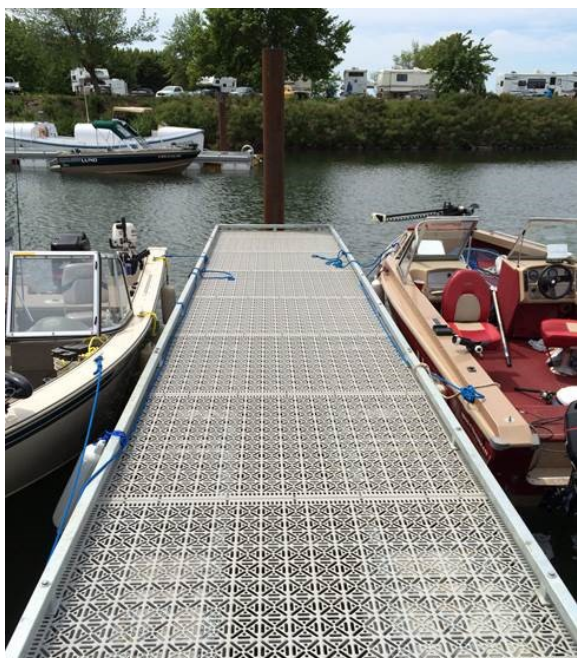
A portion of light enters the water column through deck grating and other over water structures.
