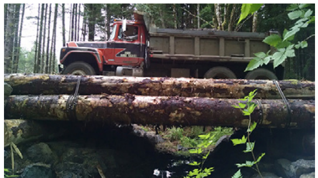
Photo 3. Log stringer bridge in the OESF.
