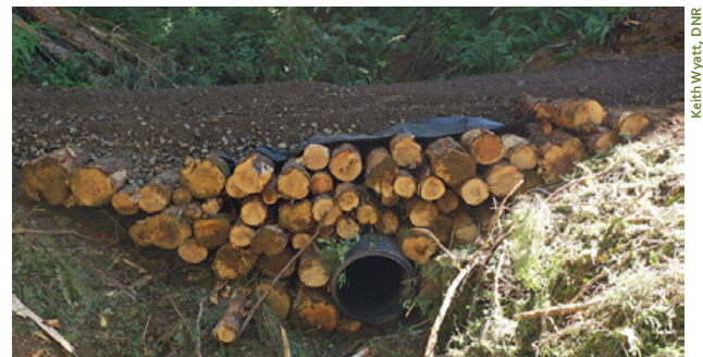
Photo 5. Temporary culvert and log fill.
