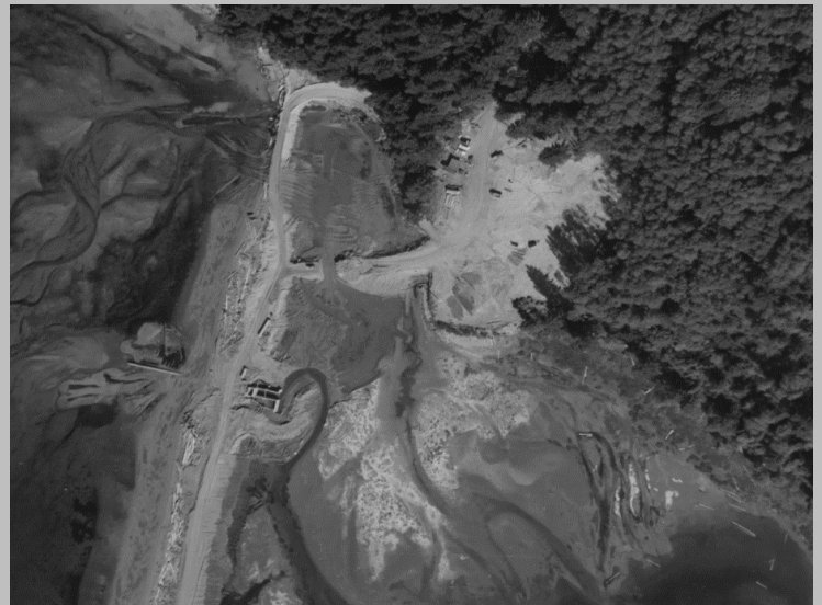
Whiteman Cove after construction of fish barrier, 1961
