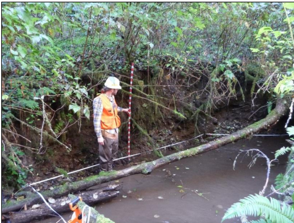
Figure 13. Field crew measuring active erosion in basin 489.
