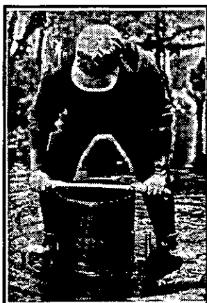
Figure 12. Force cylinder into gravel.
