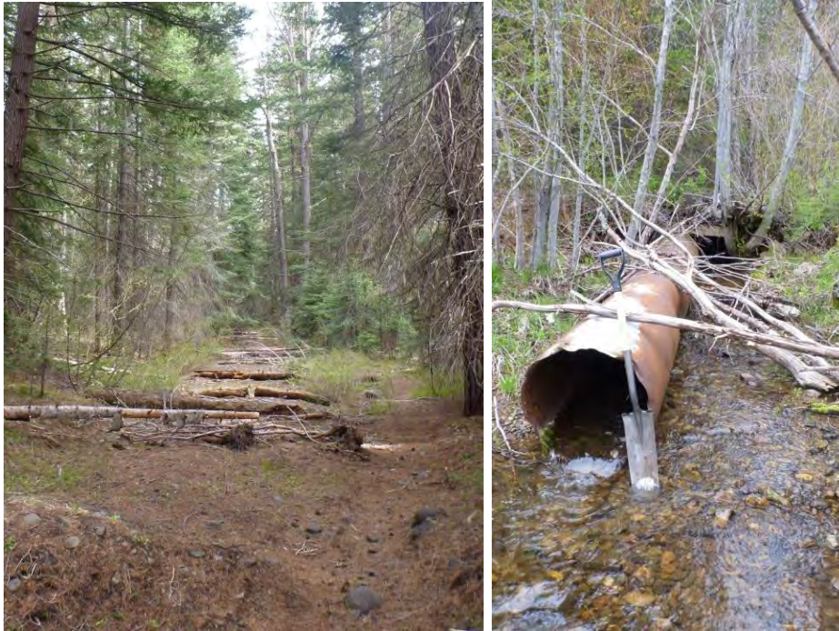
Figure 15. Wetland Improvement Opportunity 3. View of tank-trapped road and exposed culvert at its southern end.
